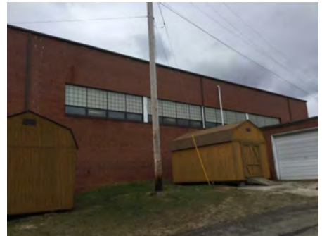
3). North Elevation - Feb 02, 2017
