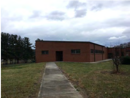
1). West Elevation - Feb 02, 2017
