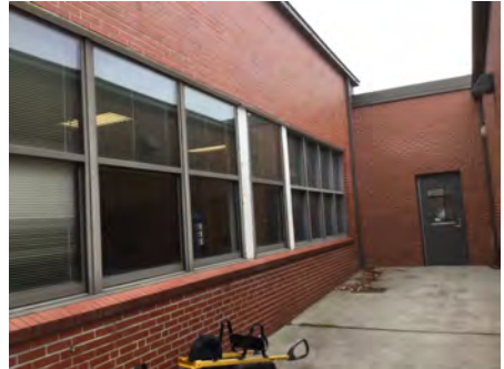
3). South Elevation - Feb 02, 2017
