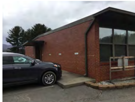
2). West Elevation - Feb 02, 2017
