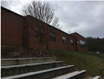
4). North Elevation - Feb 02, 2017
