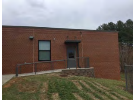
2). East Elevation - Feb 02, 2017
