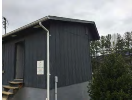
2). East Elevation - Feb 02, 2017
