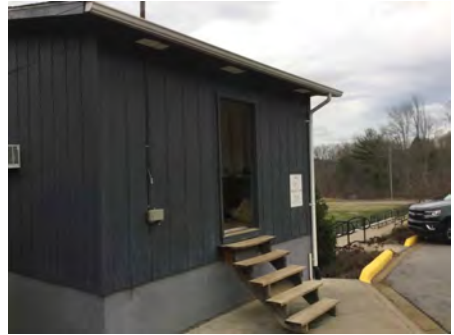
3). South Elevation - Feb 02, 2017
