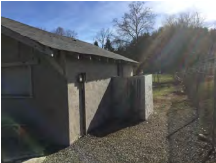
4). West Elevation - Feb 02, 2017
