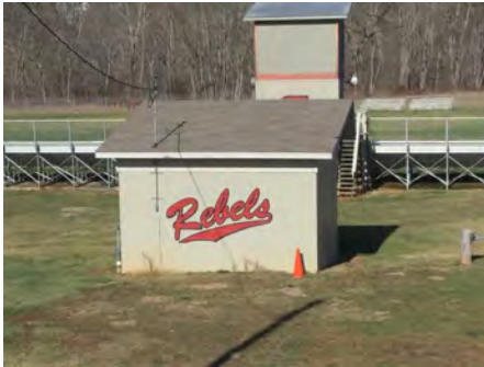
4). South Elevation - Feb 02, 2017
