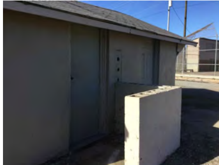
2). East Elevation - Feb 02, 2017
