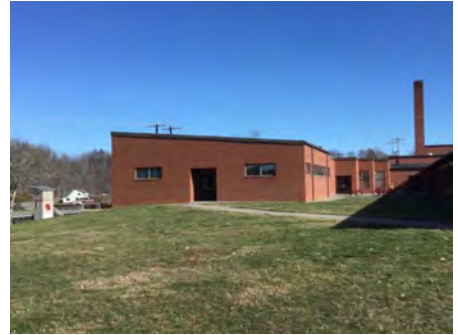
3). West Elevation - Feb 02, 2017
