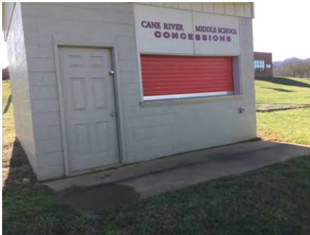
1). North Elevation - Feb 02, 2017
