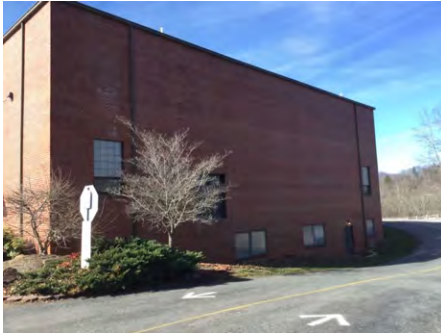
1). East Elevation - Feb 02, 2017
