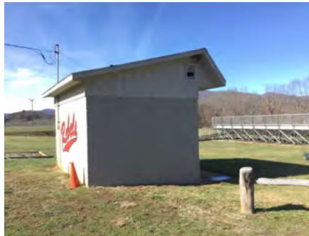
2). East Elevation - Feb 02, 2017
