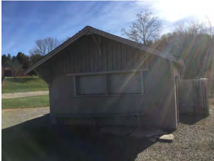
1). North Elevation - Feb 02, 2017
