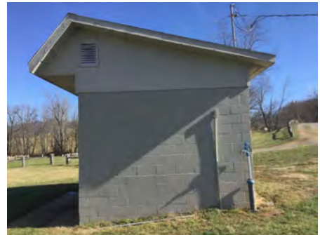
3). West Elevation - Feb 02, 2017
