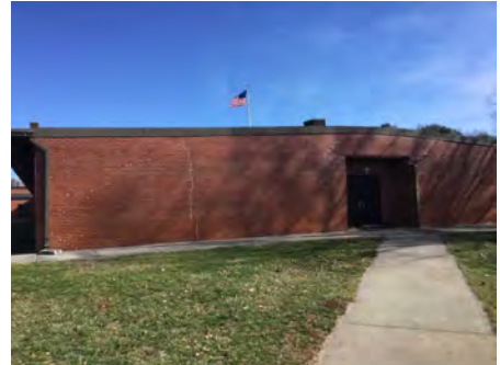
3). West Elevation - Feb 02, 2017
