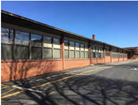
4). South Elevation - Feb 02, 2017
