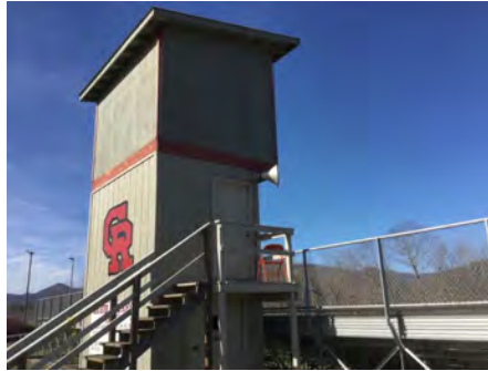
2). Southeast Elevation - Feb 02, 2017
