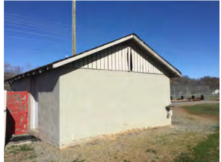
3). South Elevation - Feb 02, 2017
