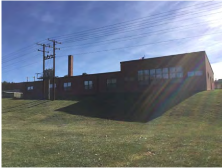
1). North Elevation - Feb 02, 2017
