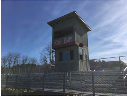
1). Northwest Elevation - Feb 02, 2017
