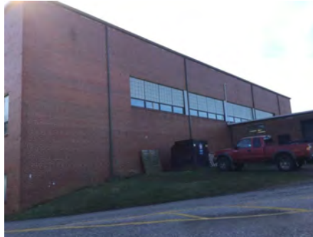
2). North Elevation - Feb 02, 2017
