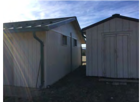
3). North Elevation - Feb 01, 2017
