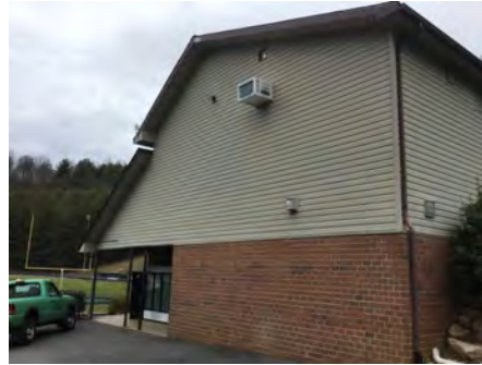
2). West Elevation - Feb 01, 2017
