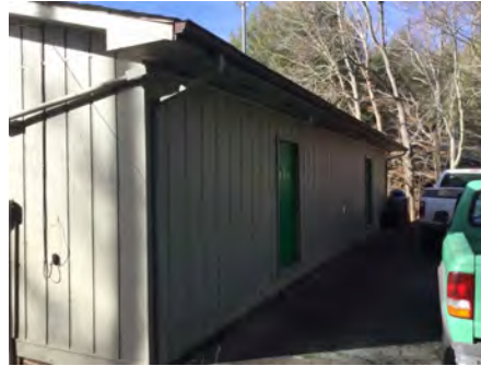
2). East Elevation - Feb 01, 2017
