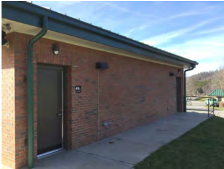
4). Southeast Elevation - Feb 01, 2017
