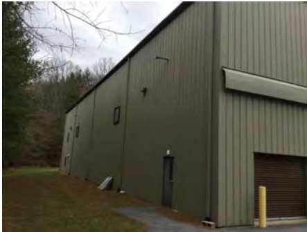
4). Southwest Elevation - Feb 01, 2017
