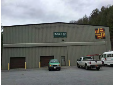
1). Southeast Elevation - Feb 01, 2017
