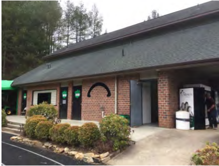
1). North Elevation - Feb 01, 2017
