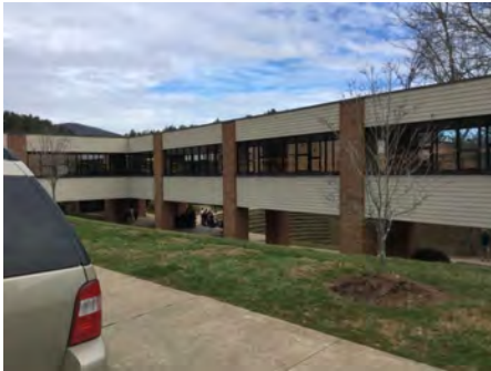
4). West Elevation - Feb 01, 2017
