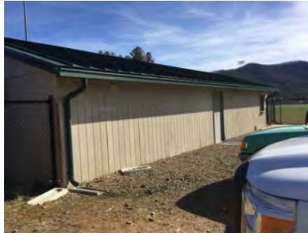
2). West Elevation - Feb 01, 2017
