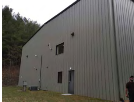
2). Northwest Elevation - Feb 01, 2017
