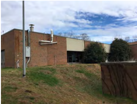
4). East Elevation - Feb 01, 2017
