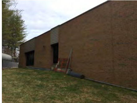
2). West Elevation - Feb 01, 2017
