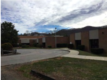
1). North Elevation - Feb 01, 2017
