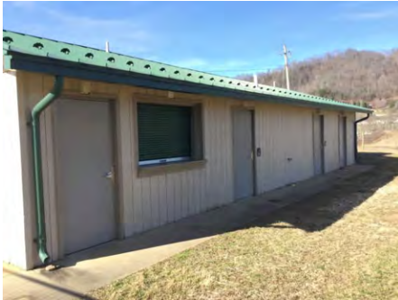
1). East Elevation - Feb 01, 2017
