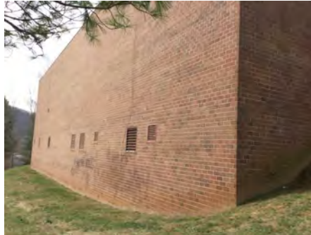
2). East Elevation - Feb 01, 2017
