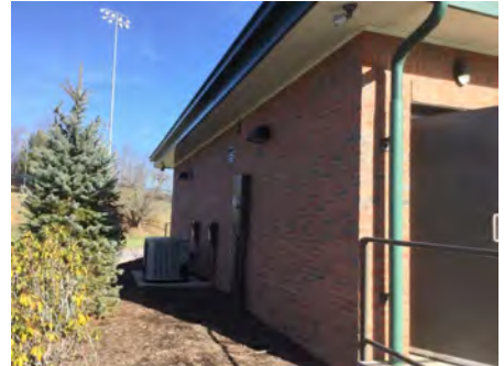
3). Northwest Elevation - Feb 01, 2017
