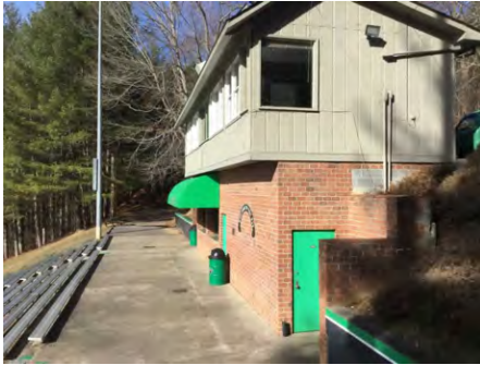
1). Southwest Elevation - Feb 01, 2017
