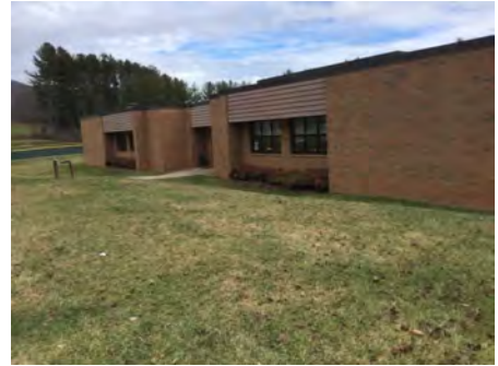
3). West Elevation - Feb 01, 2017
