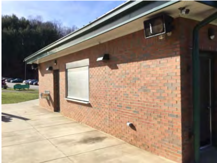
1). Southwest Elevation - Feb 01, 2017
