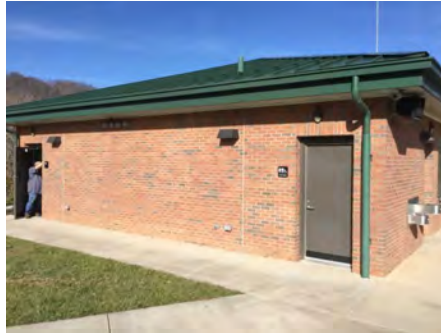
2). Southwest Elevation - Feb 01, 2017
