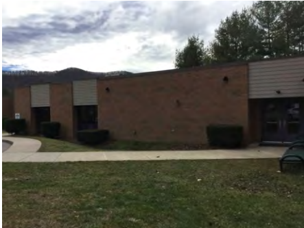
1). North Elevation - Feb 01, 2017
