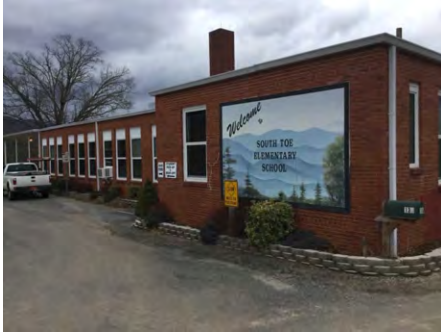
1). South Elevation - Feb 01, 2017
