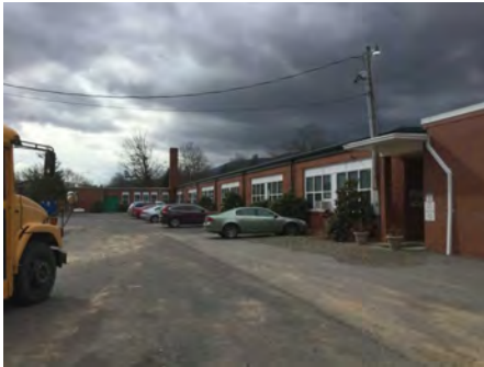
4). East Elevation - Feb 01, 2017
