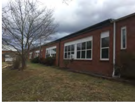
2). West Elevation - Feb 01, 2017
