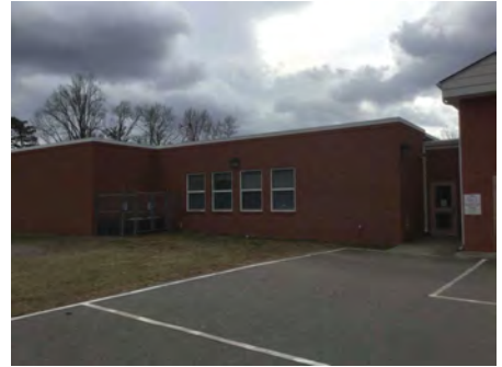
3). North Elevation - Feb 01, 2017
