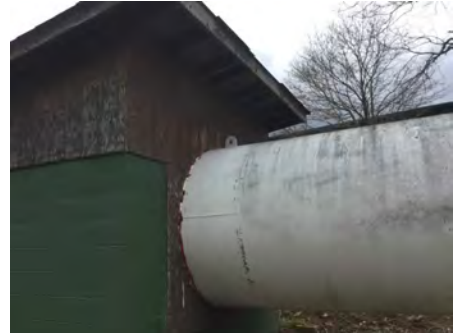
3). West Elevation - Feb 01, 2017
