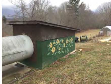
2). East Elevation - Feb 01, 2017
