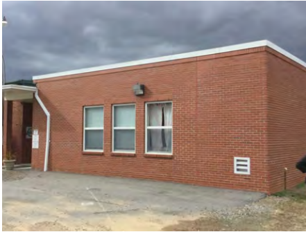
1). East Elevation - Feb 01, 2017
