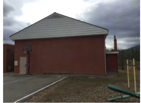
3). North Elevation - Feb 01, 2017
