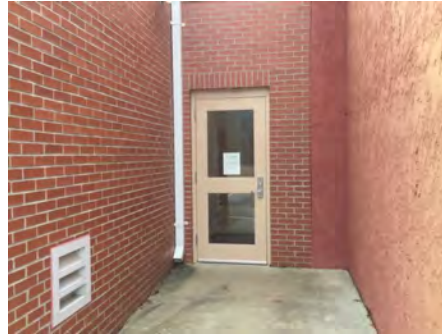
2). North Elevation - Feb 01, 2017
