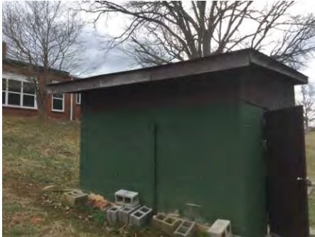
1). North Elevation - Feb 01, 2017
