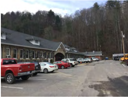
1). North Elevation - Feb 01, 2017
