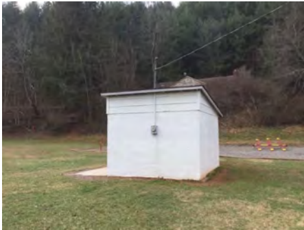
4). North Elevation - Feb 01, 2017
