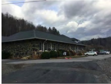
2). East Elevation - Feb 01, 2017
