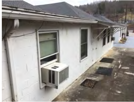
2). South Elevation - Feb 01, 2017
