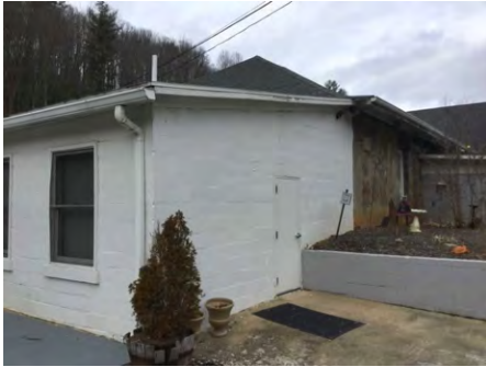
1). East Elevation - Feb 01, 2017
