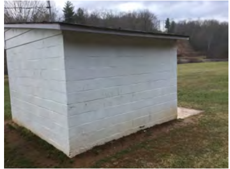
3). West Elevation - Feb 01, 2017
