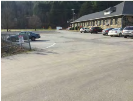
4). West Elevation - Feb 01, 2017
