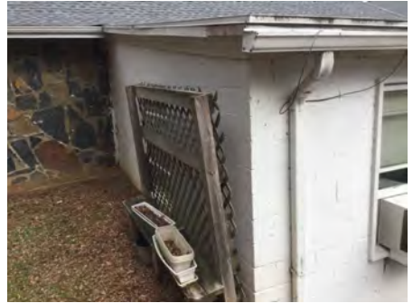
3). West Elevation - Feb 01, 2017
