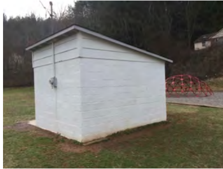
2). East Elevation - Feb 01, 2017
