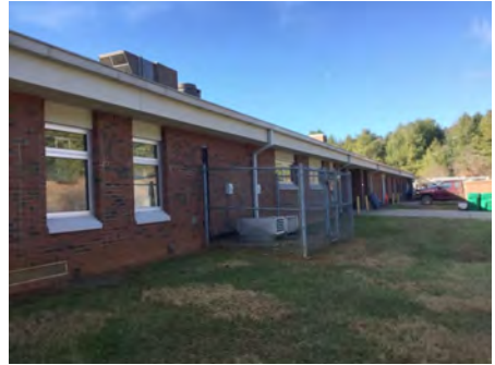
3). North Elevation - Feb 01, 2017
