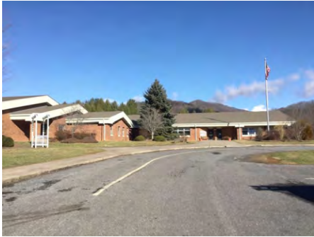
1). South Elevation - Feb 01, 2017
