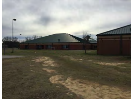
2). North Elevation - Jan 11, 2017
