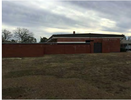
2). North Elevation - Jan 11, 2017
