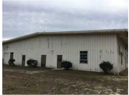
3). North Elevation - Jan 11, 2017
