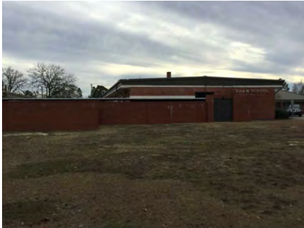
1). North Elevation - Jan 11, 2017
