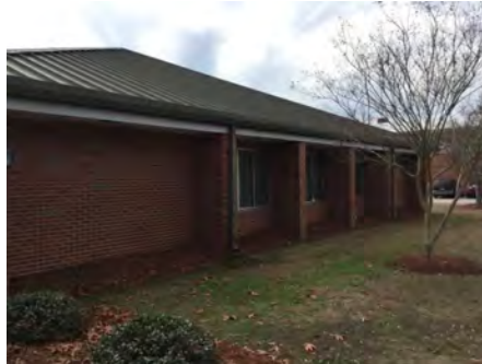
2). North Elevation - Jan 11, 2017
