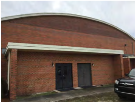
4). North Elevation - Jan 11, 2017
