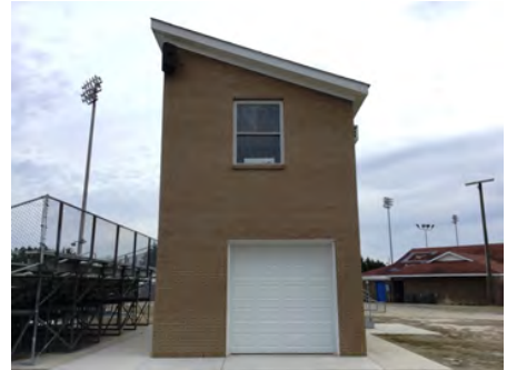
3). Southwest Elevation - Jan 12, 2017
