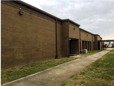
1). West Elevation - Feb 13, 2017
