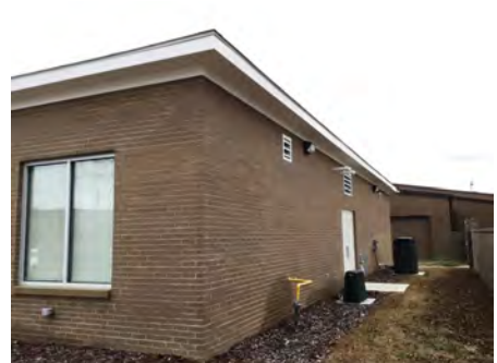
3). North Elevation - Jan 13, 2017
