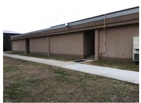
3). Southwest Elevation - Feb 14, 2017
