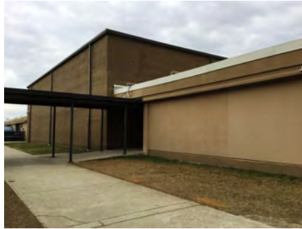
2). West Elevation - Feb 14, 2017
