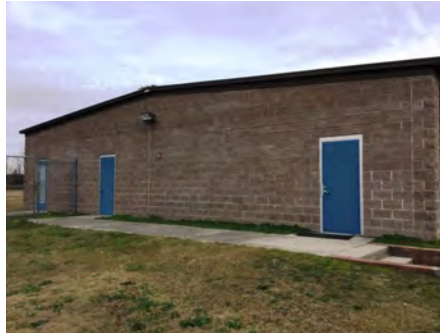
2). North Elevation - Jan 11, 2017
