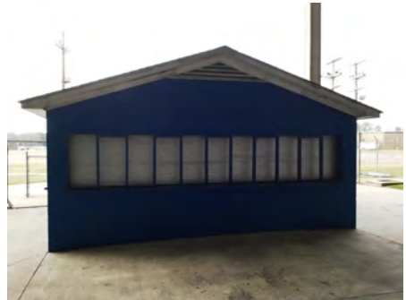
3). North Elevation - Jan 10, 2017
