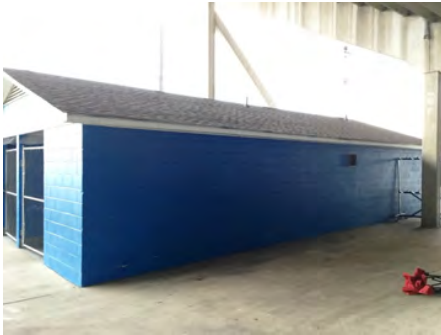
4). North Elevation - Jan 10, 2017
