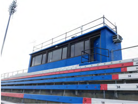
1). North Elevation - Jan 10, 2017
