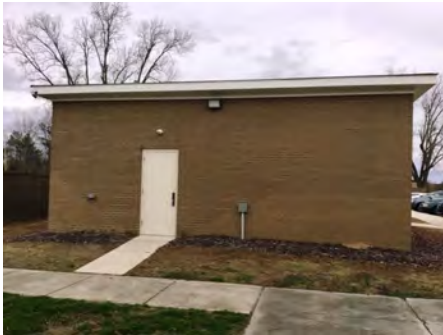
4). Southwest Elevation - Jan 13, 2017
