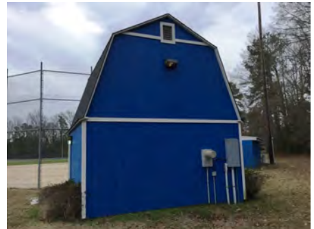
3). North Elevation - Jan 12, 2017
