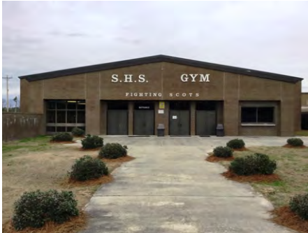
1). Southwest Elevation - Jan 11, 2017
