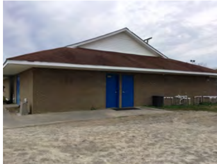
2). North Elevation - Jan 11, 2017
