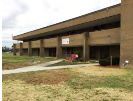
2). Southwest Elevation - Jan 11, 2017
