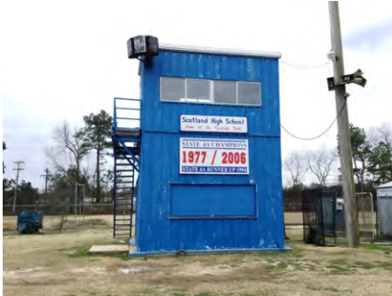
1). North Elevation - Jan 11, 2017
