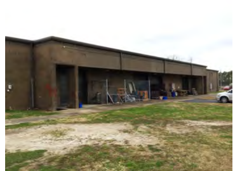
3). North Elevation - Feb 13, 2017
