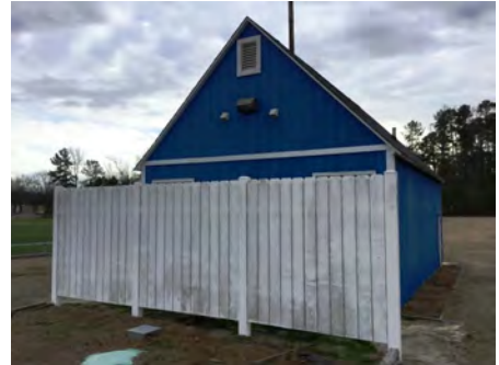
3). North Elevation - Jan 12, 2017
