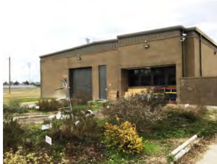
2). Northwest Elevation - Feb 13, 2017
