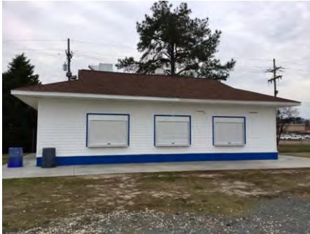
1). North Elevation - Jan 12, 2017
