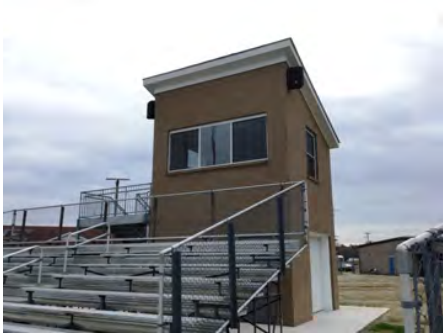
4). Northwest Elevation - Jan 12, 2017
