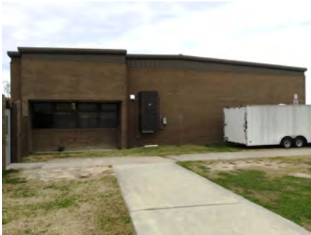
4). East Elevation - Feb 13, 2017
