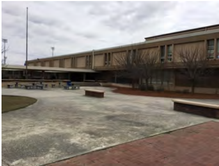
4). North Elevation - Jan 11, 2017
