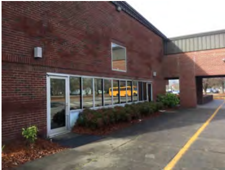
4). North Elevation - Jan 11, 2017
