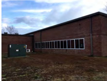
2). North Elevation - Jan 11, 2017
