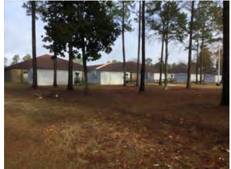
3). South Elevation - Feb 15, 2017
