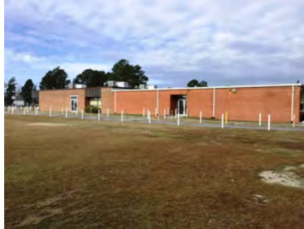
2). South Elevation - Feb 10, 2017
