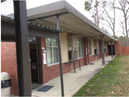
1). North Elevation - Jan 06, 2017
