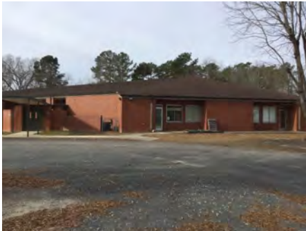
4). North Elevation - Jan 10, 2017
