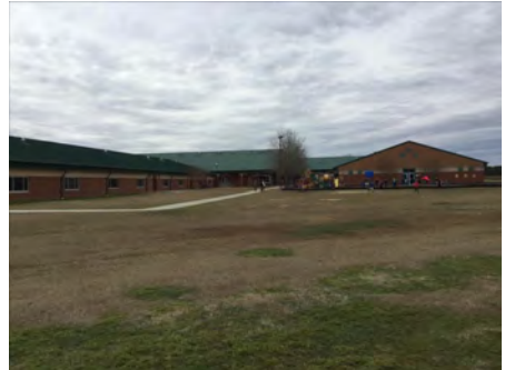
3). North Elevation - Jan 11, 2017
