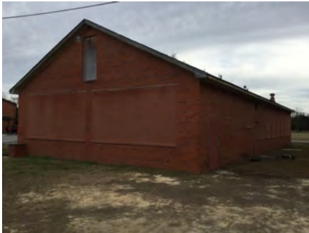
4). Northeast Elevation - Jan 10, 2017
