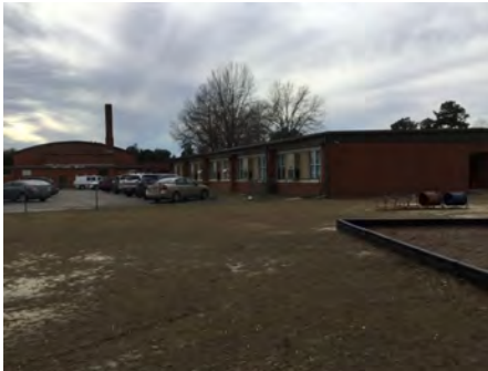
4). North Elevation - Jan 12, 2017
