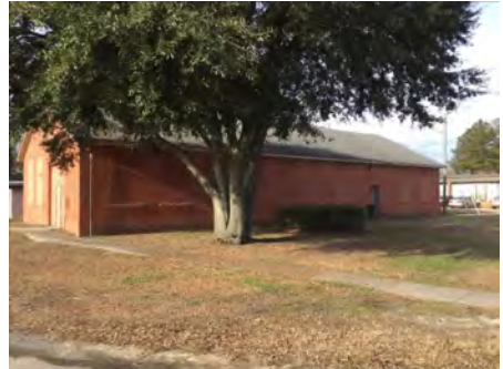
3). West Elevation - Feb 21, 2017
