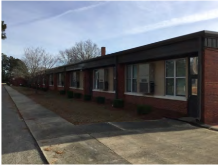
1). Northwest Elevation - Jan 10, 2017
