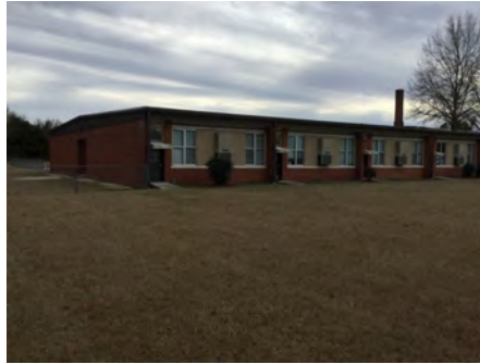
2). Northeast Elevation - Jan 10, 2017
