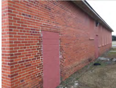
2). East Elevation - Feb 21, 2017
