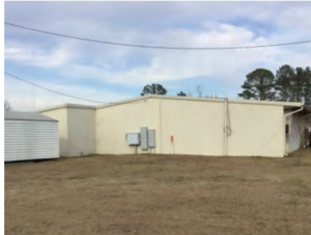
2). Southwest Elevation - Feb 16, 2017
