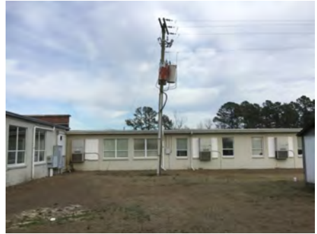
3). Southeast Elevation - Feb 16, 2017
