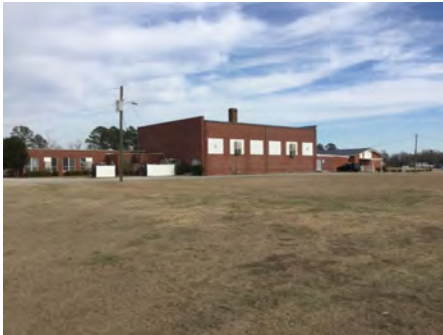
4). Southwest Elevation - Feb 16, 2017
