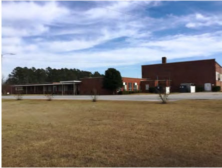
1). Northwest Elevation - Feb 16, 2017
