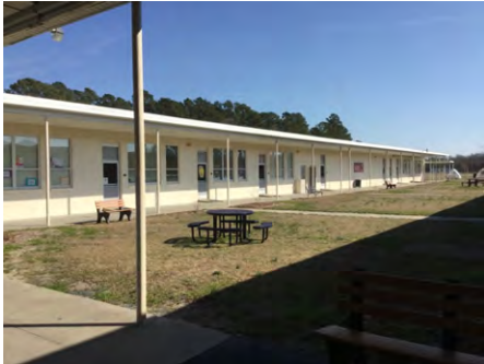
1). Northwest Elevation - Feb 16, 2017
