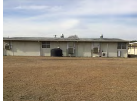
3). Southeast Elevation - Feb 16, 2017
