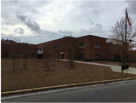
1). North Elevation - Dec 07, 2016
