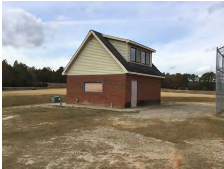
1). North Elevation - Dec 07, 2016
