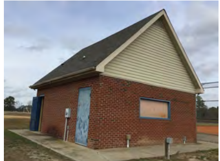
3). South Elevation - Dec 07, 2016
