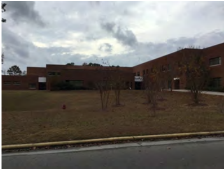
4). East Elevation - Dec 07, 2016
