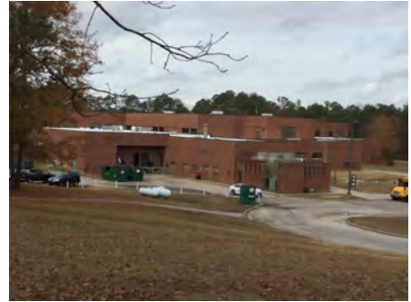
3). South Elevation - Dec 07, 2016
