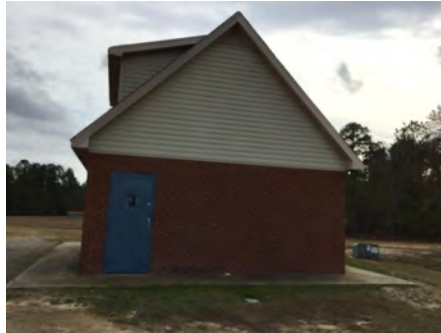
2). West Elevation - Dec 07, 2016
