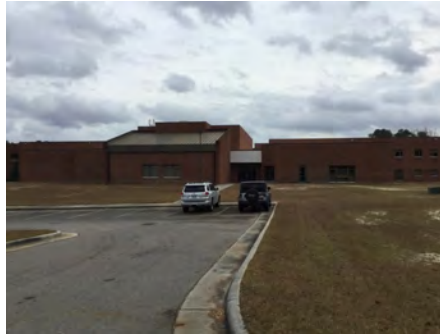
2). West Elevation - Dec 07, 2016
