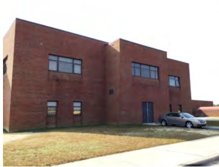
2). Northeast Elevation - Nov 15, 2016
