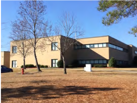
1). Northeast Elevation - Dec 06, 2016
