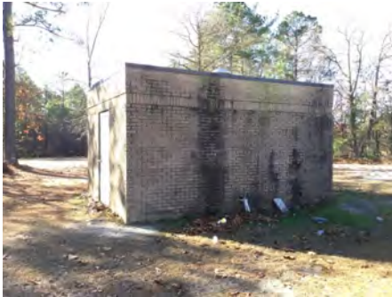
4). West Elevation - Dec 06, 2016
