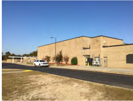
2). West Elevation - Dec 06, 2016
