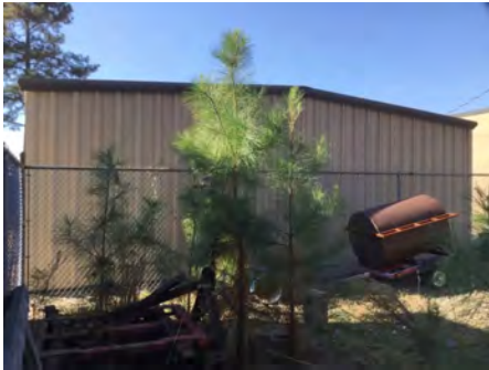
4). East Elevation - Dec 06, 2016
