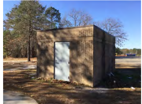
3). North Elevation - Dec 06, 2016
