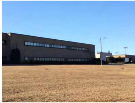
5). North Elevation - Dec 06, 2016
