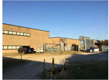
3). South Elevation - Dec 06, 2016
