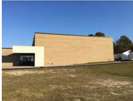
2). West Elevation - Dec 06, 2016
