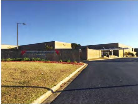
1). Northwest Elevation - Dec 06, 2016
