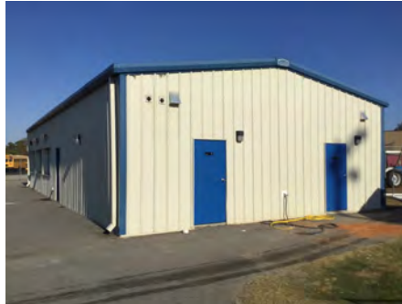
2). Southwest Elevation - Nov 21, 2016
