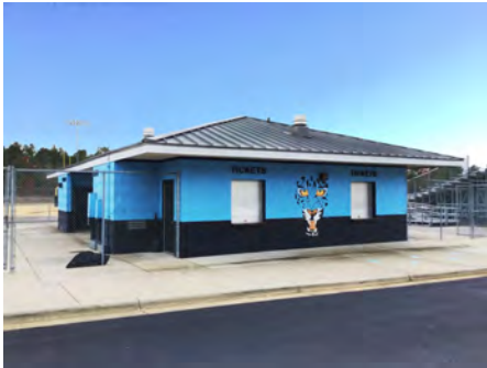
4). Northeast Elevation - Dec 08, 2016
