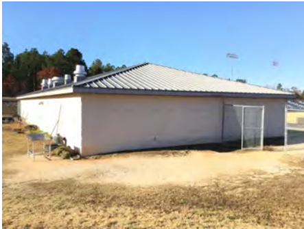
4). Northeast Elevation - Dec 08, 2016
