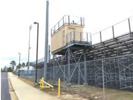
4). Northwest Elevation - Dec 08, 2016
