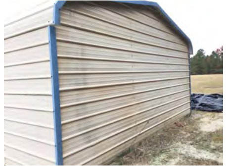
3). Northwest Elevation - Dec 08, 2016
