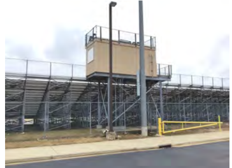
3). Northeast Elevation - Dec 08, 2016
