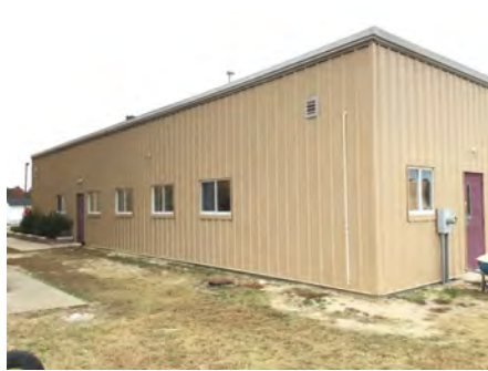
2). East Elevation - Dec 08, 2016
