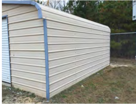
2). Northeast Elevation - Dec 08, 2016
