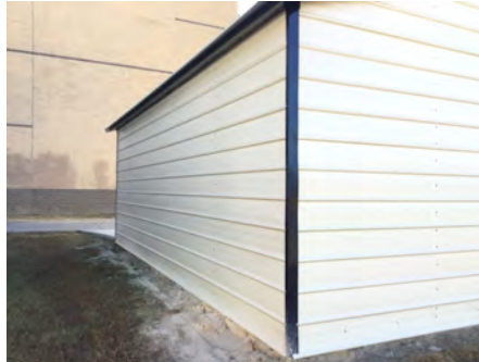
2). North Elevation - Dec 08, 2016
