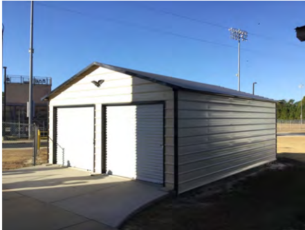
1). East Elevation - Dec 08, 2016
