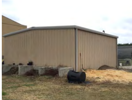
2). North Elevation - Dec 08, 2016
