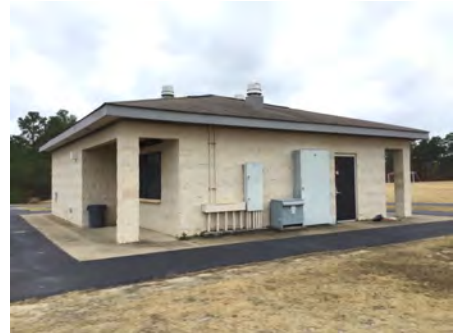
3). North Elevation - Dec 08, 2016
