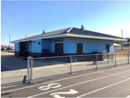
1). Northwest Elevation - Dec 08, 2016
