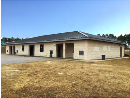
1). Northwest Elevation - Dec 08, 2016
