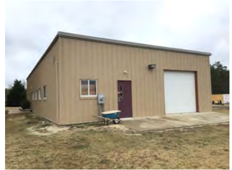
3). North Elevation - Dec 08, 2016
