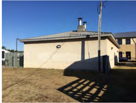
2). South Elevation - Dec 08, 2016
