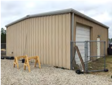
4). South Elevation - Dec 08, 2016
