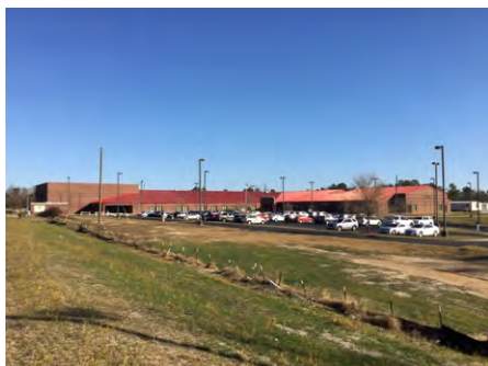
1). Southwest Elevation - Dec 01, 2016
