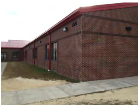
8). Northeast Elevation - Nov 28, 2016
