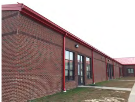
7). Northeast Elevation - Nov 28, 2016
