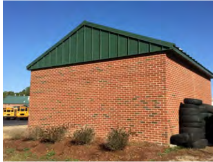
2). South Elevation - Dec 06, 2016
