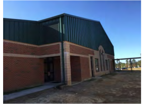
3). North Elevation - Dec 06, 2016
