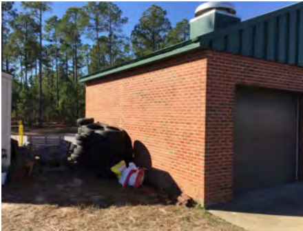
4). East Elevation - Dec 06, 2016
