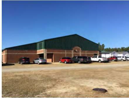
2). East Elevation - Dec 06, 2016
