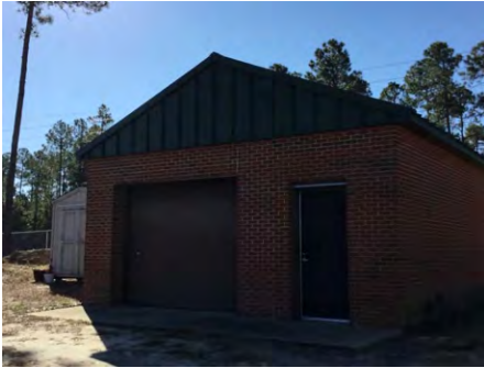
1). North Elevation - Dec 06, 2016
