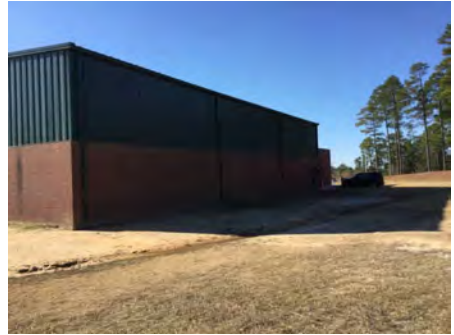
3). North Elevation - Dec 06, 2016
