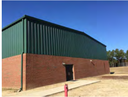
2). East Elevation - Dec 06, 2016
