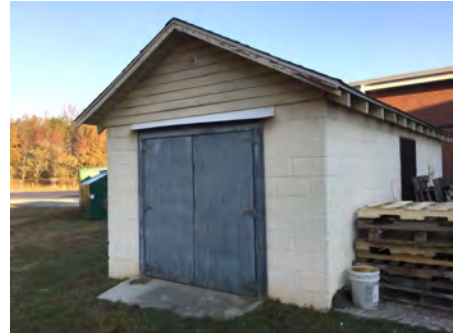
3). South Elevation - Dec 08, 2016
