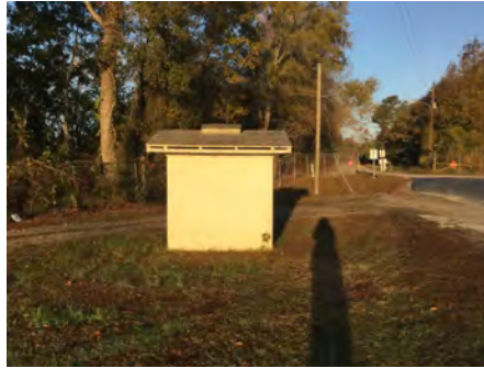
2). North Elevation - Dec 08, 2016
