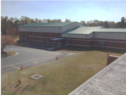
1). North Elevation - Dec 08, 2016
