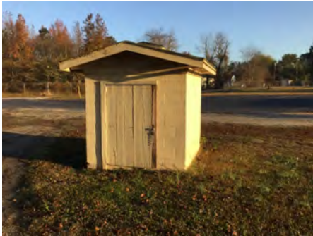
4). South Elevation - Dec 08, 2016
