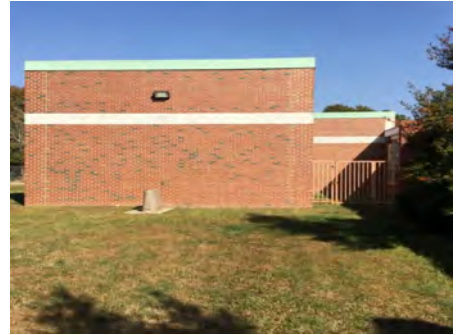
3). South Elevation - Dec 08, 2016
