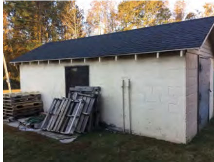
2). East Elevation - Dec 08, 2016
