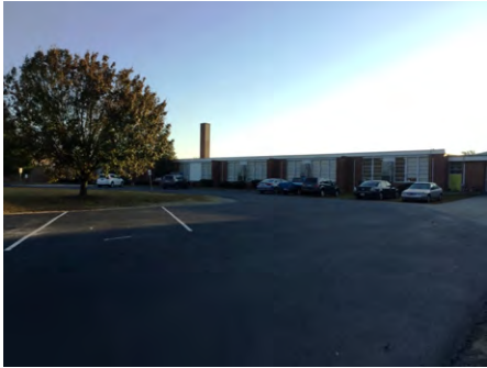
1). West Elevation - Dec 09, 2016
