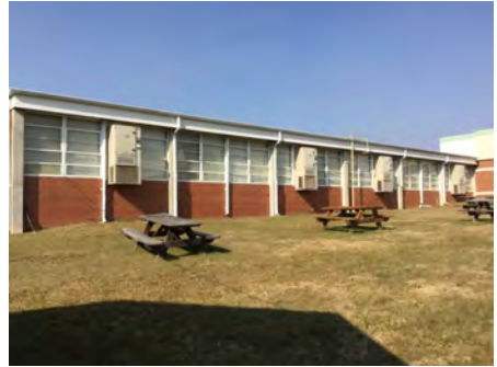
3). East Elevation - Dec 09, 2016
