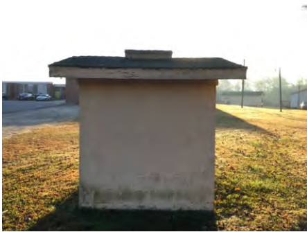
1). West Elevation - Dec 08, 2016
