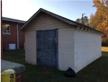
1). North Elevation - Dec 08, 2016
