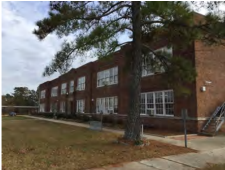
4). North Elevation - Dec 02, 2016
