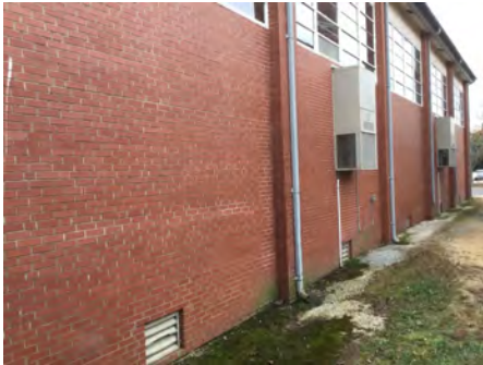
4). North Elevation - Dec 06, 2016
