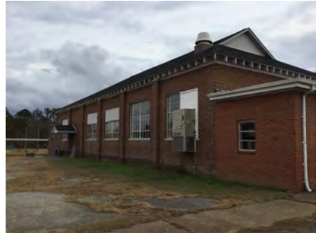
3). North Elevation - Dec 06, 2016
