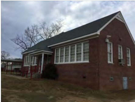
4). South Elevation - Dec 02, 2016
