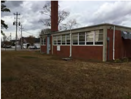
4). East Elevation - Dec 02, 2016
