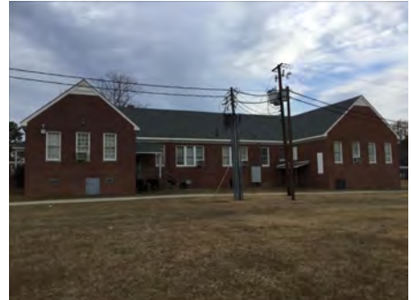
3). East Elevation - Dec 02, 2016
