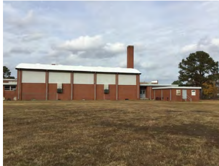
2). South Elevation - Dec 06, 2016
