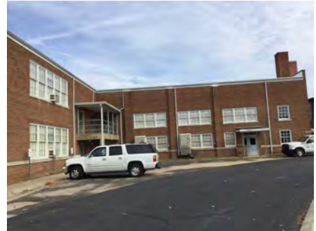
3). East Elevation - Dec 02, 2016
