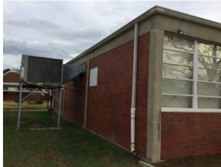
2). North Elevation - Dec 02, 2016
