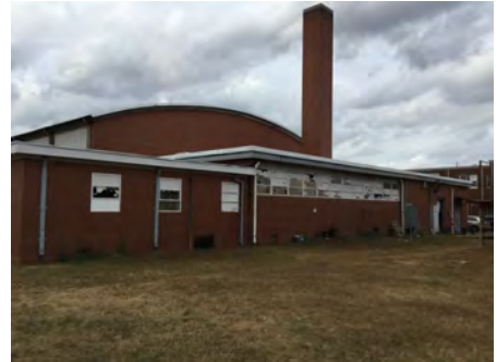
3). East Elevation - Dec 02, 2016
