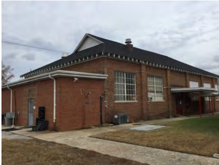
1). South Elevation - Dec 02, 2016
