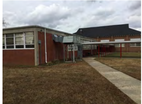
3). South Elevation - Dec 02, 2016
