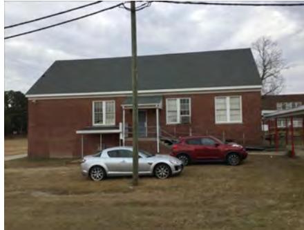
2). North Elevation - Dec 02, 2016
