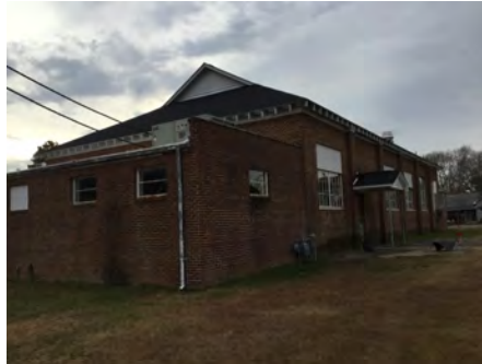
2). East Elevation - Dec 06, 2016
