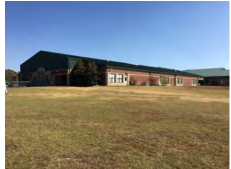
6). Southwest Elevation - Nov 29, 2016
