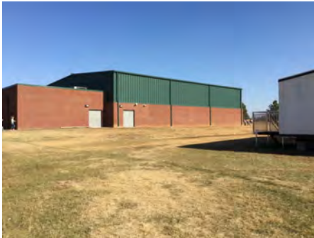
4). Southwest Elevation - Nov 22, 2016
