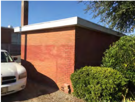
4). South Elevation - Dec 06, 2016
