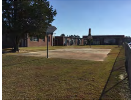
2). North Elevation - Dec 06, 2016
