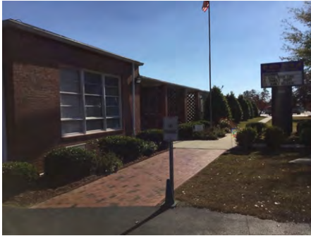
1). East Elevation - Dec 06, 2016
