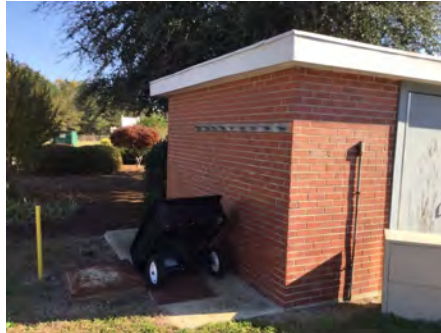
2). North Elevation - Dec 06, 2016
