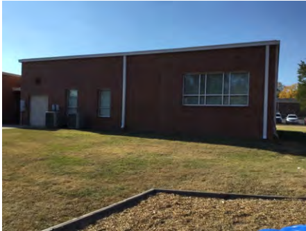
1). East Elevation - Dec 06, 2016
