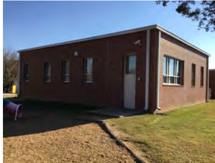
2). North Elevation - Dec 06, 2016
