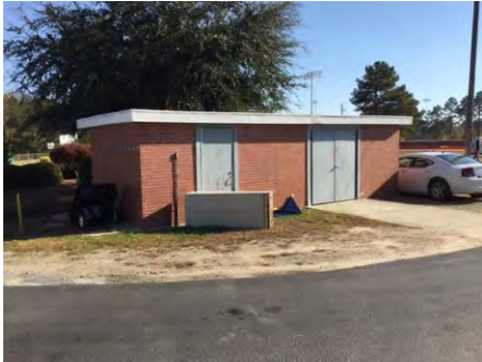
1). East Elevation - Dec 06, 2016
