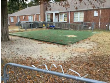
1). North Elevation - Dec 06, 2016
