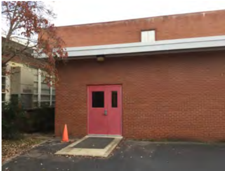
4). North Elevation - Dec 06, 2016
