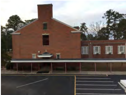
4). South Elevation - Dec 06, 2016
