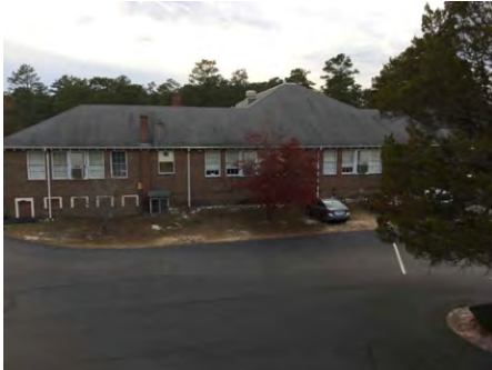
1). North Elevation - Mar 06, 2017
