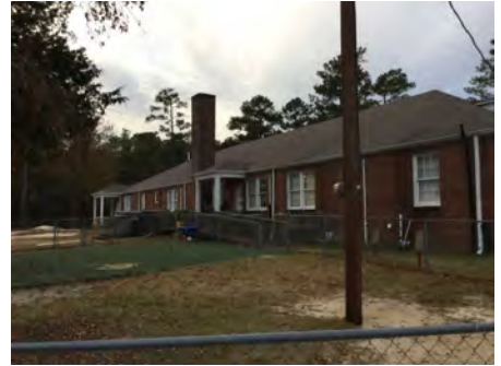
3). South Elevation - Dec 06, 2016
