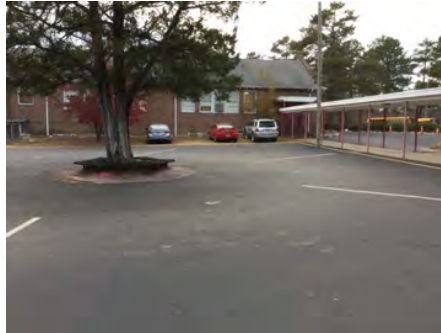
2). East Elevation - Mar 06, 2017
