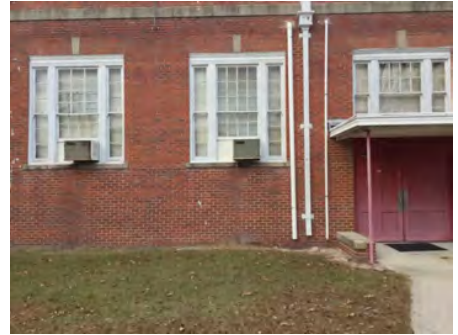
3). South Elevation - Dec 06, 2016
