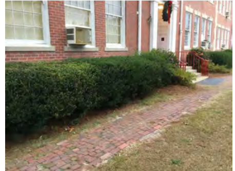
3). West Elevation - Dec 06, 2016
