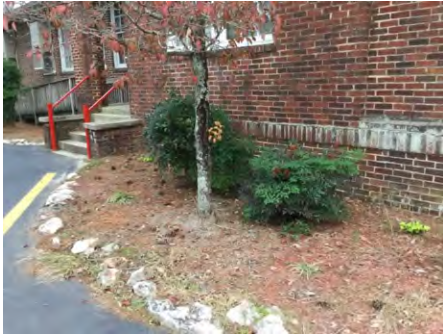
1). North Elevation - Dec 06, 2016
