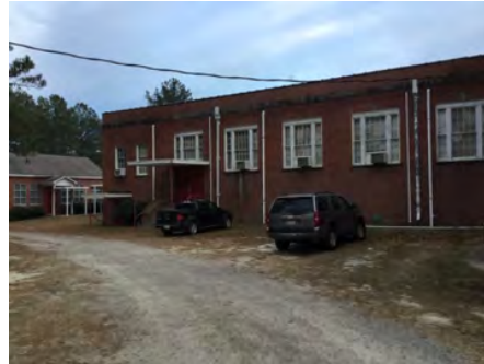
2). North Elevation - Dec 06, 2016
