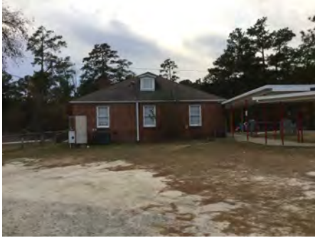
4). East Elevation - Dec 06, 2016
