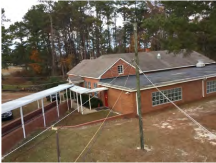
1). West Elevation - Dec 06, 2016
