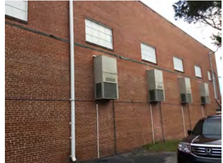
3). East Elevation - Dec 06, 2016
