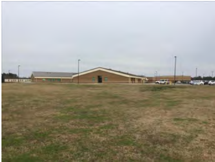
4). North Elevation - Feb 22, 2017
