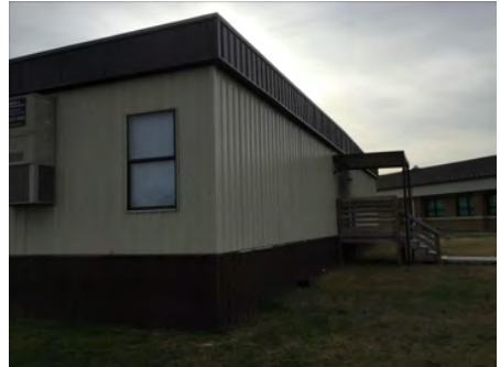
3). West Elevation - Feb 22, 2017
