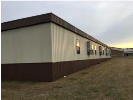
4). South Elevation - Feb 22, 2017
