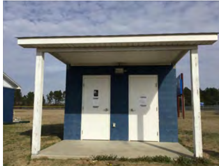
2). North Elevation - Feb 22, 2017
