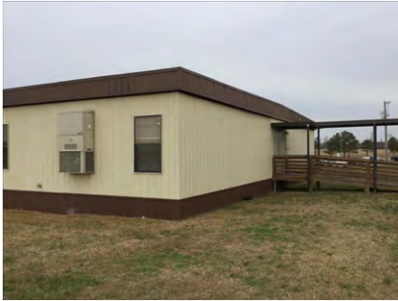
1). East Elevation - Feb 22, 2017
