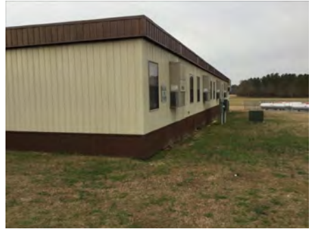
3). North Elevation - Feb 22, 2017
