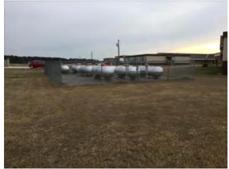
3). East Elevation - Feb 22, 2017
