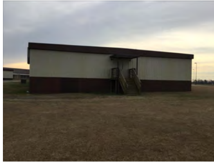
2). West Elevation - Feb 22, 2017
