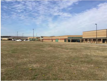
1). South Elevation - Feb 22, 2017
