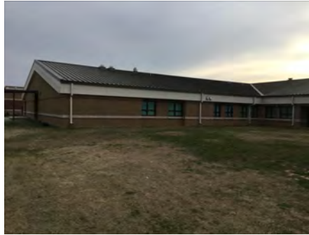
2). West Elevatrion - Feb 22, 2017
