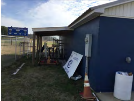
4). North Elevation - Feb 22, 2017
