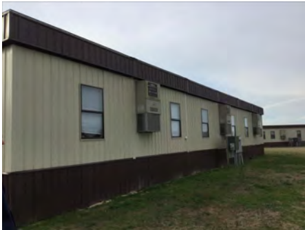
4). North Elevation - Feb 22, 2017
