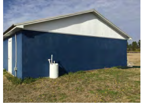
3). West Elevation - Feb 22, 2017
