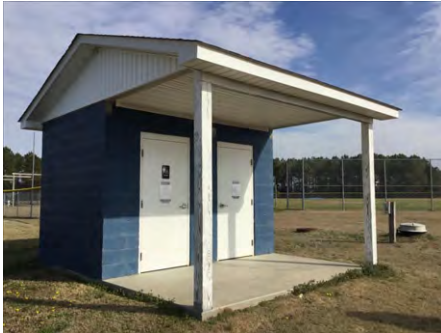
1). Northwest Elevation - Feb 22, 2017
