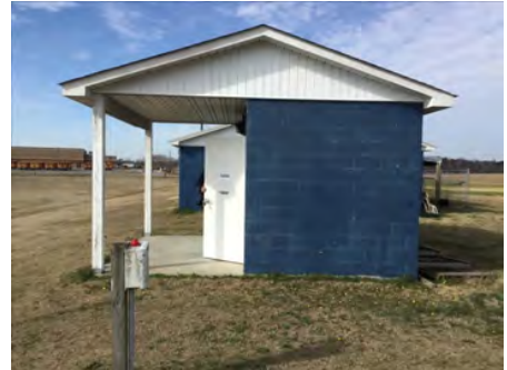
3). East Elevation - Feb 22, 2017
