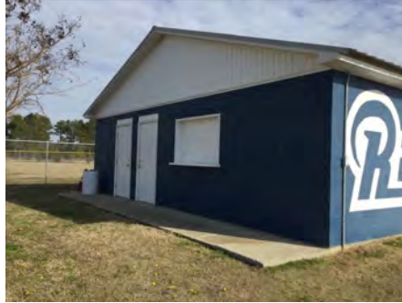
2). East Elevation - Feb 22, 2017
