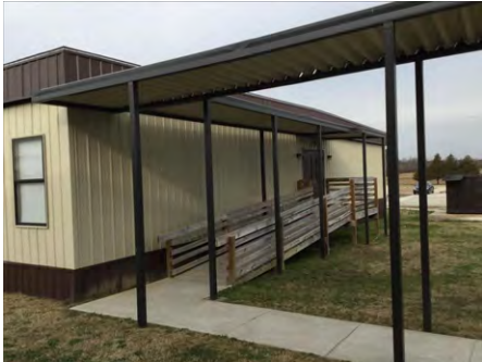
1). East Elevation - Feb 22, 2017
