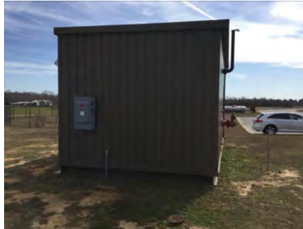
2). North Elevation - Feb 21, 2017
