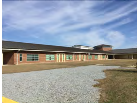
2). Southeast Elevation - Feb 21, 2017
