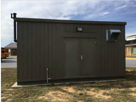
1). East Elevation - Feb 21, 2017
