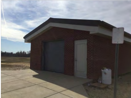
1). East Elevation - Feb 22, 2017
