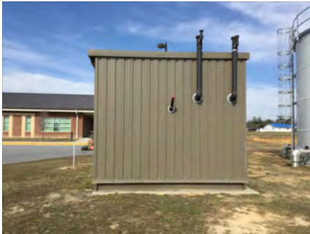
4). South Elevation - Feb 21, 2017
