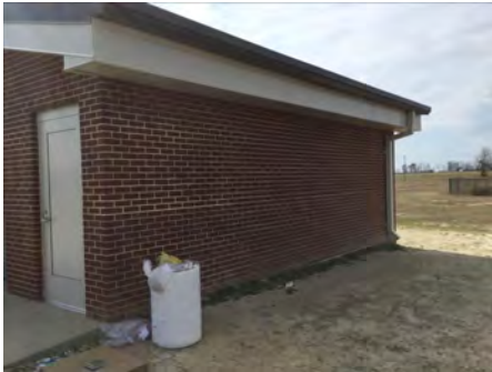
4). North Elevation - Feb 22, 2017
