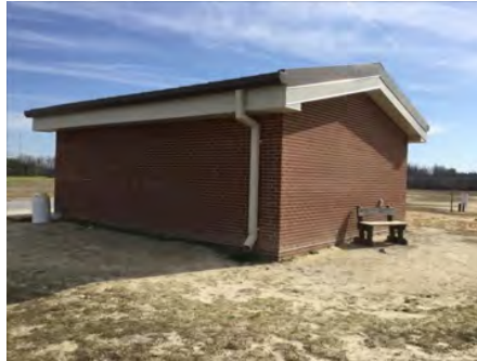
2). West Elevation - Feb 22, 2017
