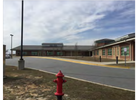
3). Southwest Elevation - Feb 21, 2017
