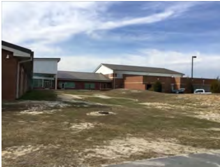
4). Northwest Elevation - Feb 21, 2017
