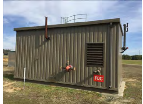
3). West Elevation - Feb 21, 2017
