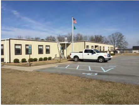
1). South Elevation - Feb 15, 2017
