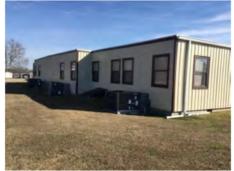
3). North Elevation - Feb 15, 2017
