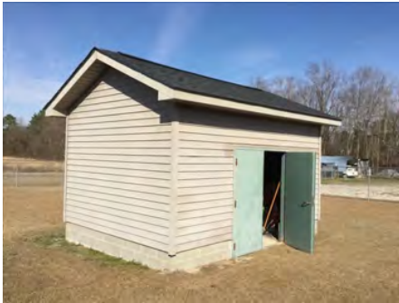
4). West Elevation - Feb 23, 2017
