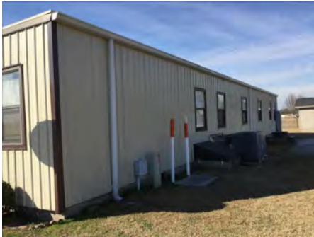
4). East Elevation - Feb 15, 2017
