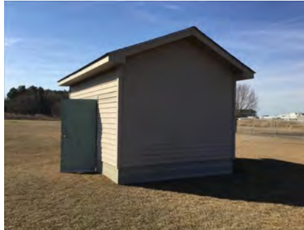
2). East Elevation - Feb 23, 2017
