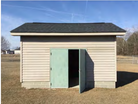
1). North Elevation - Feb 23, 2017
