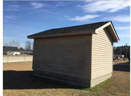
3). South Elevation - Feb 23, 2017
