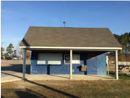
4). South Elevation - Feb 17, 2017
