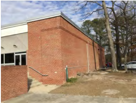
4). South Elevation - Feb 16, 2017
