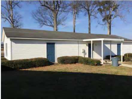
1). East Elevation - Feb 13, 2017
