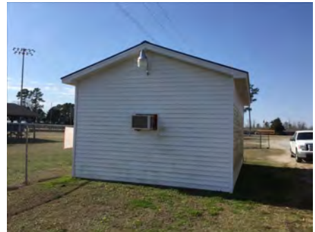
3). East Elevation - Feb 23, 2017
