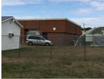
2). East Elevation - Feb 13, 2017
