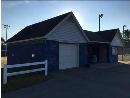
1). North Elevation - Feb 17, 2017
