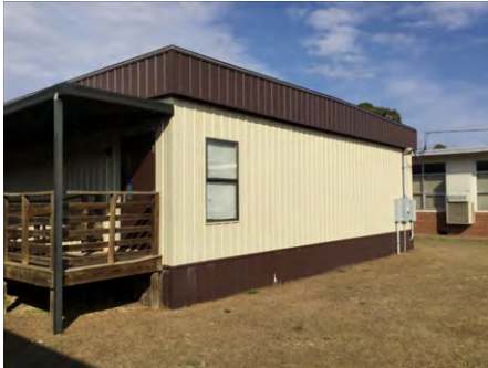
1). South Elevation - Feb 17, 2017
