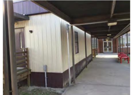
3). North Elevation - Feb 17, 2017
