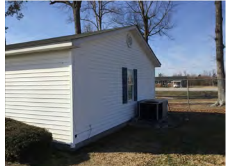
3). North Elevation - Feb 13, 2017
