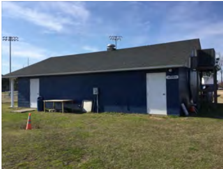
4). South Elevation - Feb 16, 2017
