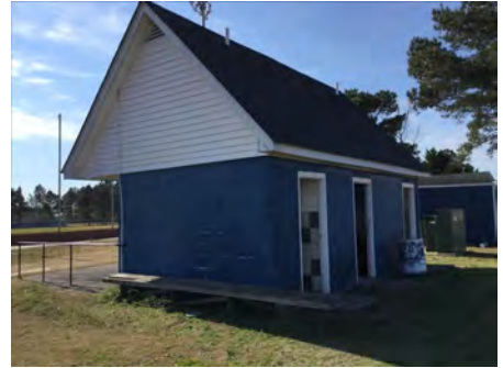
3). North Elevation - Feb 16, 2017
