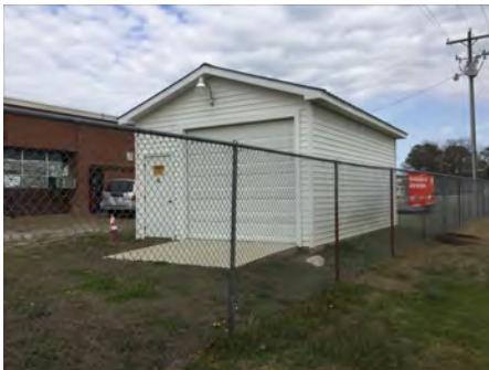
4). South Elevation - Feb 23, 2017
