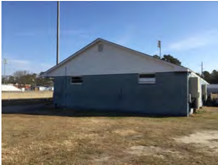
4). South Elevation - Feb 13, 2017
