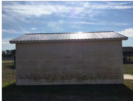
2). North Elevation - Feb 23, 2017
