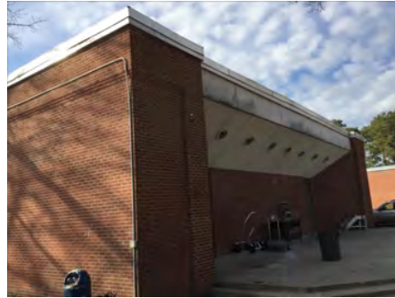
2). East Elevation - Feb 16, 2017
