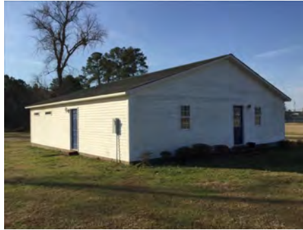
2). South Elevation - Feb 13, 2017
