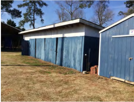
1). East Elevation - Feb 23, 2017
