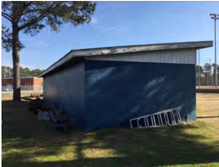
4). North Elevation - Feb 16, 2017
