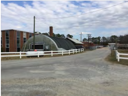
4). East Elevation - Feb 16, 2017
