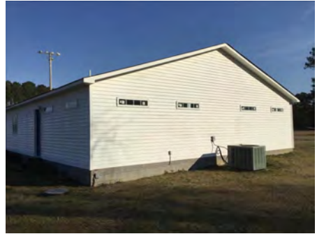
3). North Elevation - Feb 23, 2017
