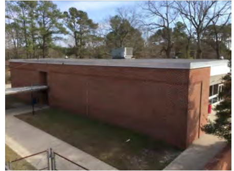
3). North Elevation - Feb 16, 2017
