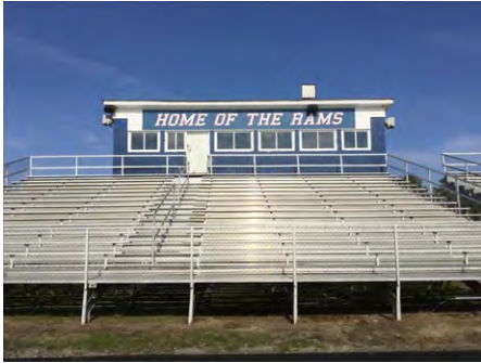
1). South Elevation - Feb 16, 2017
