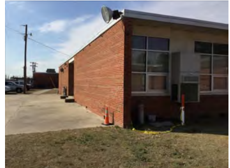
3). South Elevation - Feb 16, 2017
