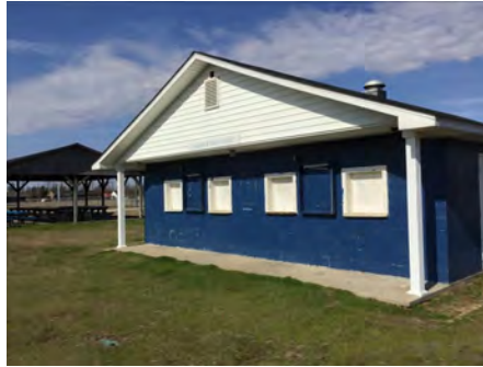
2). North Elevation - Feb 16, 2017
