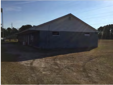
1). North Elevation - Feb 13, 2017
