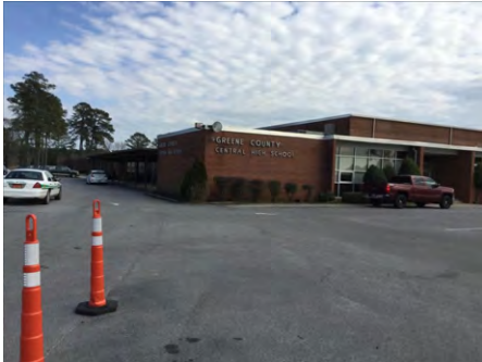
1). North Elevation - Feb 16, 2017
