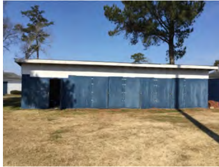
2). South Elevation - Feb 16, 2017
