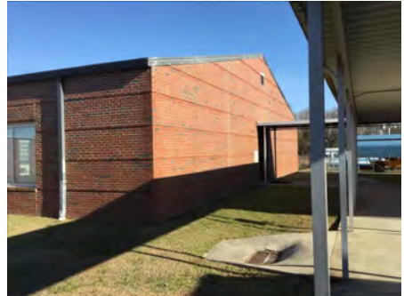
3). Southeast Elevation - Feb 13, 2017
