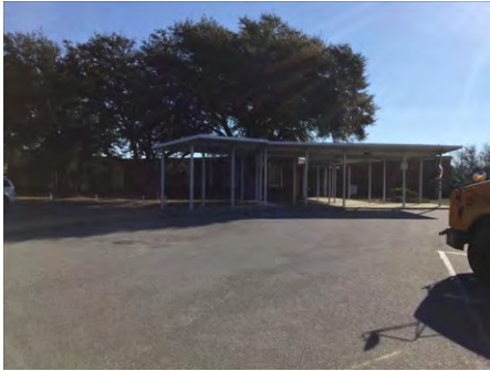
1). West Elevation - Feb 13, 2017
