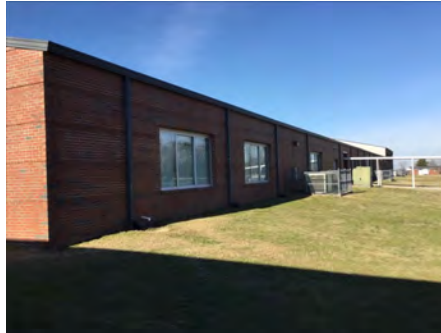
2). Northeast Elevation - Feb 13, 2017
