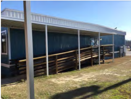
4). Southwest Elevation - Feb 13, 2017
