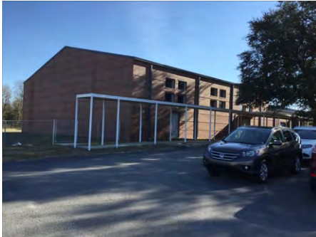
1). Northwest Elevation - Feb 13, 2017
