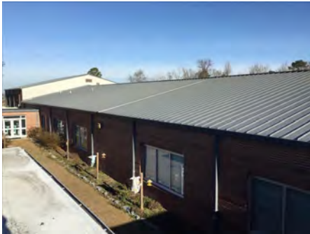
4). Northwest Elevation - Feb 13, 2017
