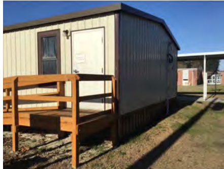
2). Northeast Elevation - Feb 13, 2017
