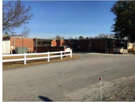
2). East Elevation - Feb 13, 2017
