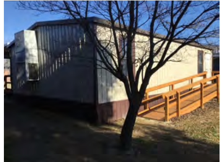
3). Southwest Elevation - Feb 13, 2017
