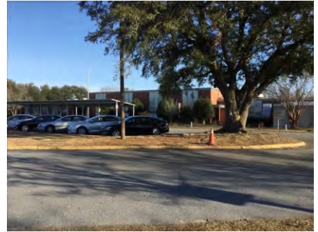
3). South Elevation - Feb 13, 2017
