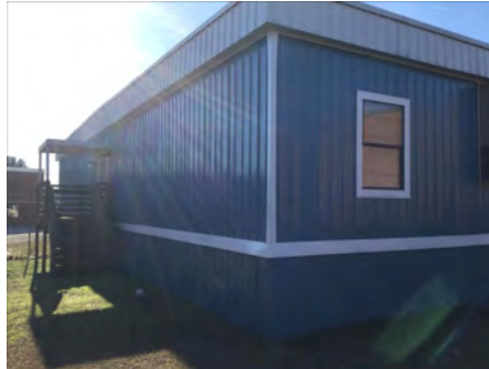
2). Northwest Elevation - Feb 13, 2017
