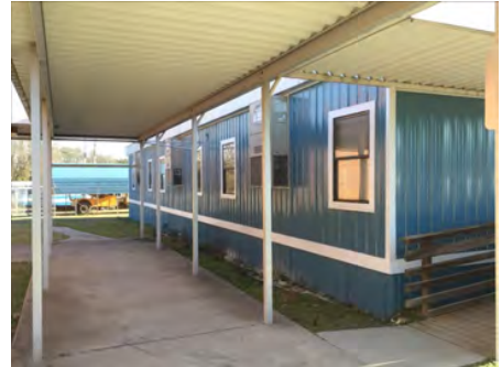
3). Southeast Elevation - Feb 13, 2017
