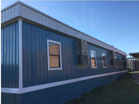
1). Northeast Elevation - Feb 13, 2017
