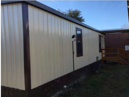
1). Northwest Elevation - Feb 13, 2017
