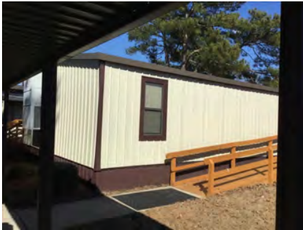
4). East Elevation - Feb 01, 2017
