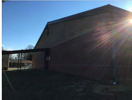
2). North Elevation - Feb 22, 2017
