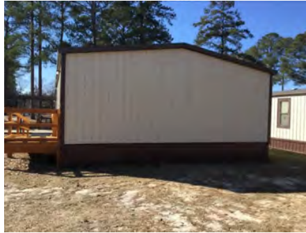
2). West Elevation - Feb 01, 2017
