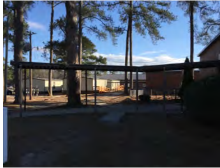
2). North Elevation - Feb 13, 2017
