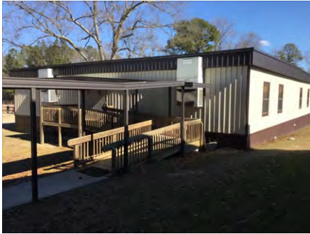
1). West Elevation - Feb 13, 2017
