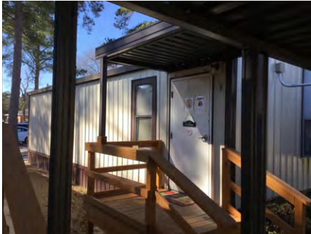
1). North Elevation - Feb 10, 2017
