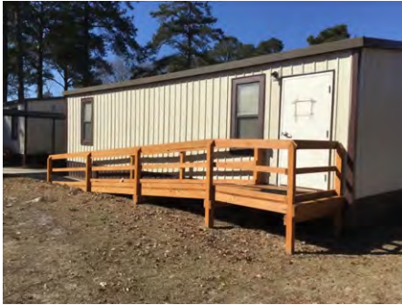
1). North Elevation - Feb 01, 2017
