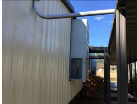
2). West Elevation - Feb 10, 2017
