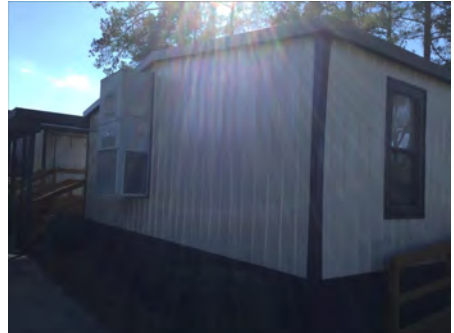
3). West Elevation - Feb 10, 2017
