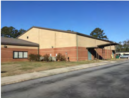
4). East Elevation - Feb 13, 2017
