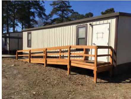
2). South Elevation - Feb 10, 2017
