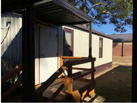
1). North Elevation - Feb 10, 2017
