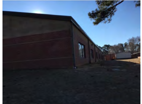
3). West Elevation - Feb 22, 2017
