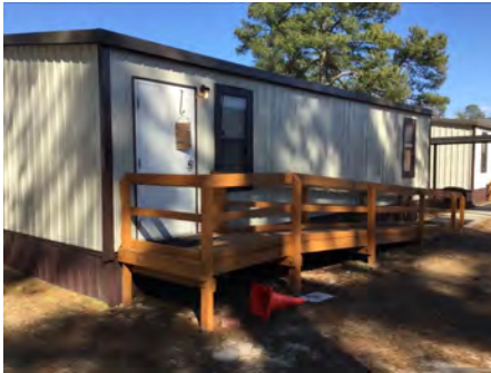
4). North Elevation - Feb 10, 2017
