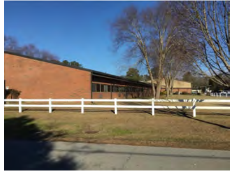
3). East Elevation - Feb 13, 2017
