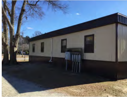
2). North Elevation - Feb 13, 2017
