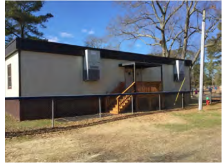
3). East Elevation - Feb 13, 2017
