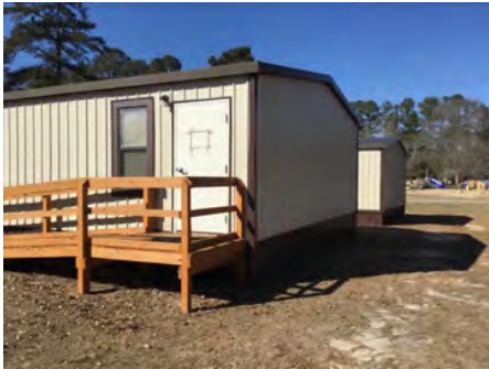
4). East Elevation - Feb 10, 2017
