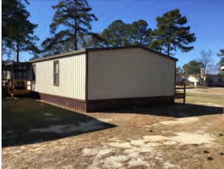
4). Southwest Elevation - Feb 01, 2017
