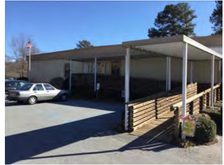
3). North Elevation - Jan 31, 2017
