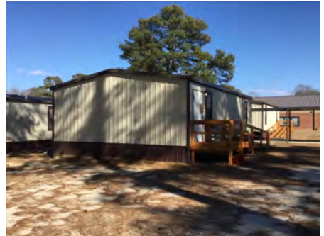
3). East Elevation - Feb 10, 2017
