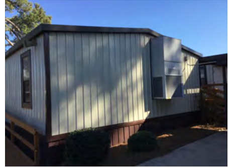
3). East Elevation - Feb 10, 2017
