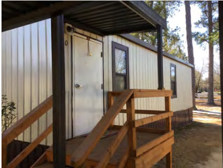
1). South Elevation - Feb 10, 2017
