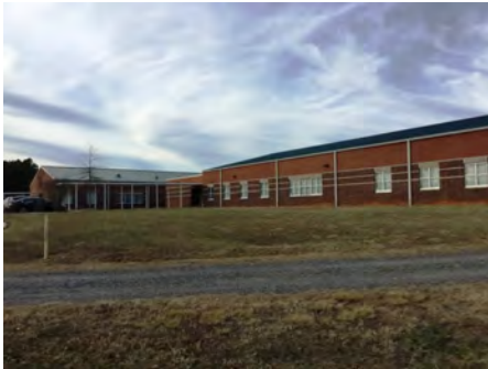
4). South Elevation - Feb 13, 2017
