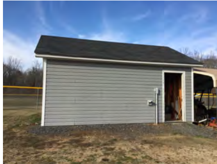
2). South Elevation - Feb 11, 2017
