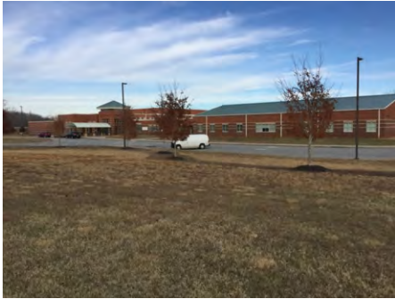
1). West Elevation - Feb 13, 2017
