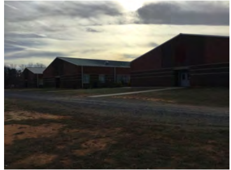
3). East Elevation - Feb 13, 2017
