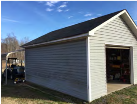
4). North Elevation - Feb 11, 2017
