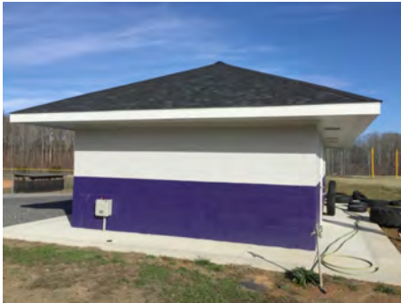
4). East Elevation - Feb 11, 2017
