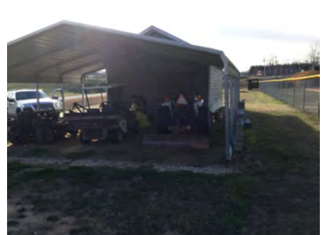
3). East Elevation - Feb 11, 2017
