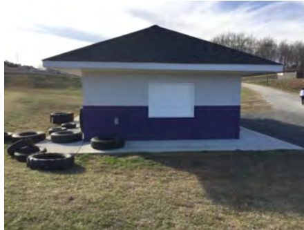
2). West Elevation - Feb 11, 2017
