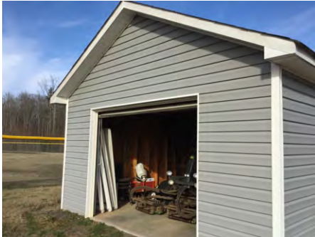
1). West Elevation - Feb 11, 2017
