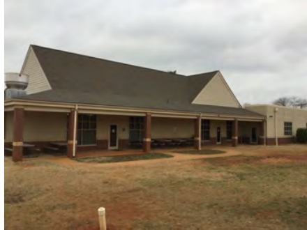
2). Southeast Elevation - Feb 14, 2017
