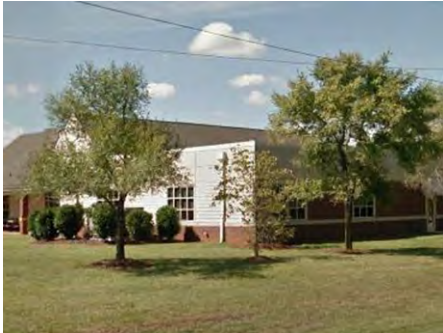
1). Southeast Elevation - Feb 14, 2017
