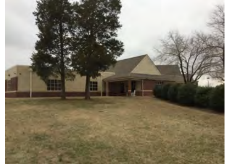
3). Northwest Elevation - Feb 14, 2017
