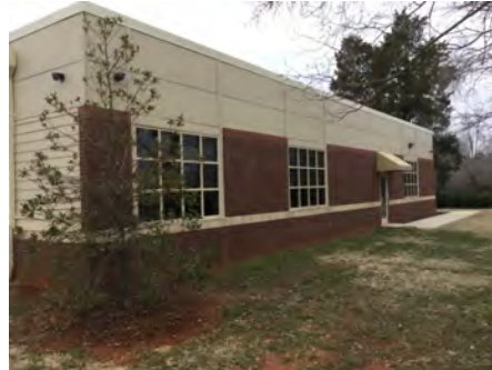
2). Northeast Elevation - Feb 14, 2017
