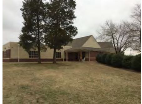
3). Northwest Elevation - Feb 14, 2017
