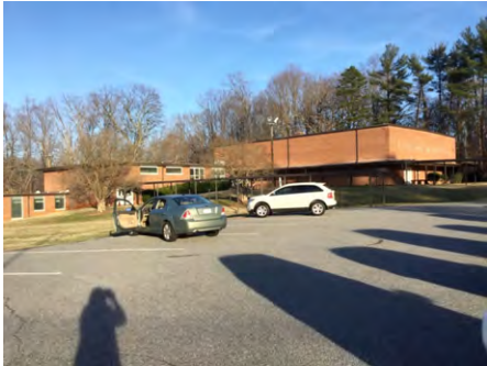
1). Southwest Elevation - Feb 14, 2017
