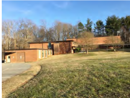
2). Northwest Elevation - Feb 14, 2017
