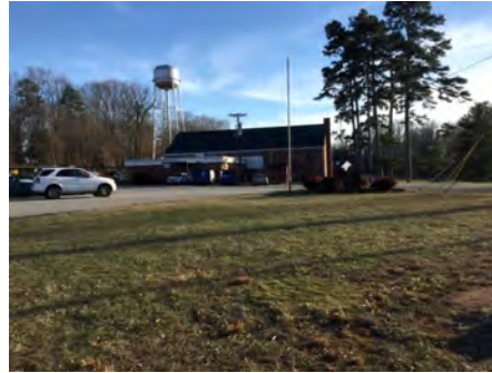
2). North Elevation - Feb 14, 2017
