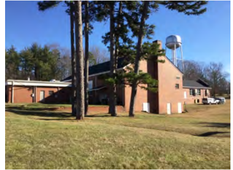
3). West Elevation - Feb 14, 2017
