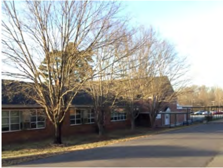
1). East Elevation - Feb 14, 2017
