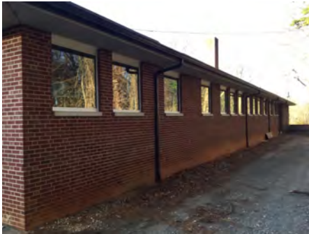
4). Southeast Elevation - Feb 14, 2017
