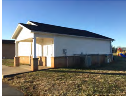
2). North Elevation - Feb 10, 2017
