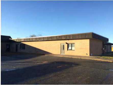
1). Northeast Elevation - Feb 10, 2017
