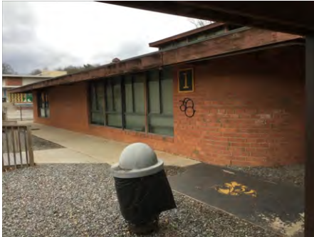
1). North Elevation - Jan 17, 2017
