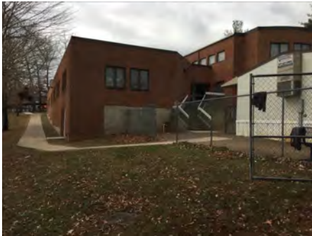
4). Northwest Elevation - Jan 23, 2017
