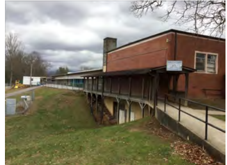
3). North Elevation - Jan 23, 2017
