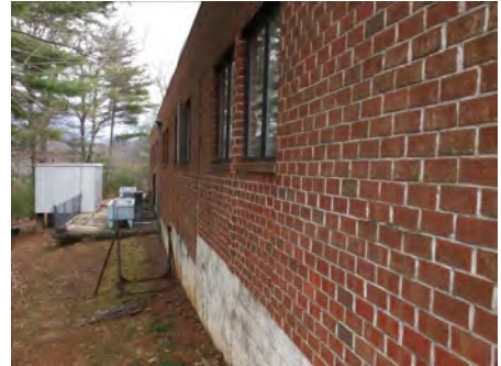
3). Northeast Elevation - Jan 23, 2017
