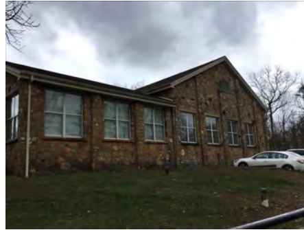
2). North Elevation - Jan 17, 2017
