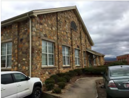
4). South Elevation - Feb 15, 2017
