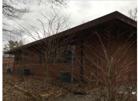
3). North Elevation - Jan 23, 2017
