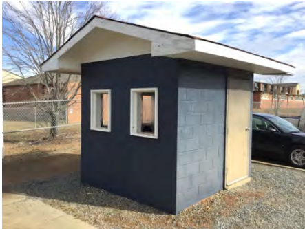
1). Southwest Elevation - Feb 15, 2017
