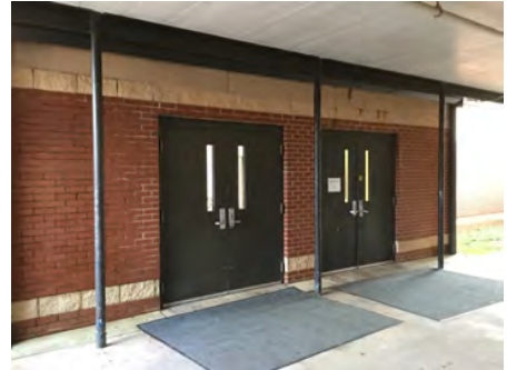
3). West Elevation - Feb 16, 2017
