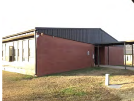
2). North Elevation - Feb 12, 2017
