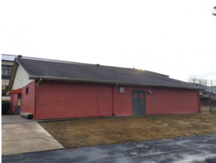
4). West Elevation - Feb 12, 2017
