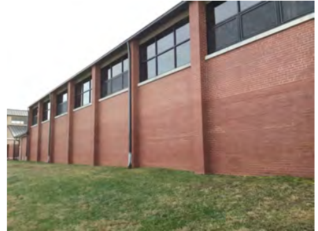
3). South Elevation - Feb 16, 2017
