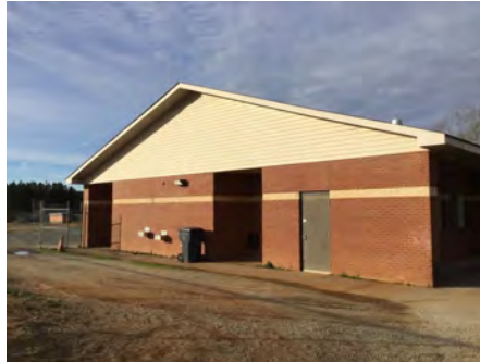
2). East Elevation - Feb 12, 2017
