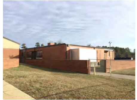
3). Southwest Elevation - Feb 16, 2017
