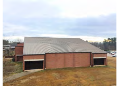
3). West Elevation - Feb 16, 2017
