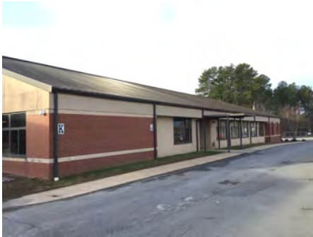
4). North Elevation - Feb 12, 2017
