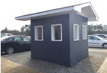
4). Northwest Elevation - Feb 15, 2017
