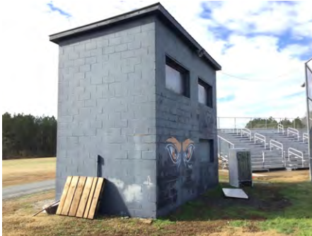
1). Northeast Elevation - Feb 15, 2017
