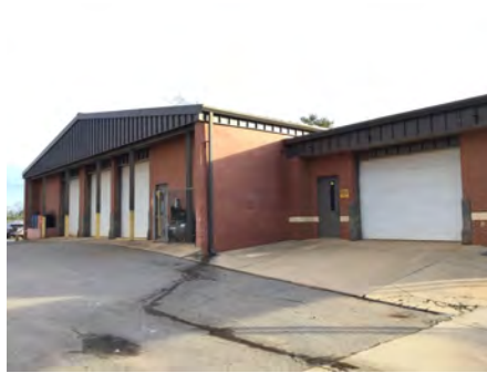
2). West Elevation - Feb 12, 2017
