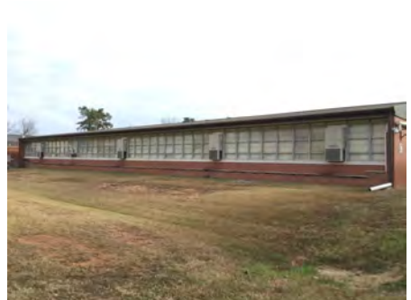
3). West Elevation - Feb 12, 2017
