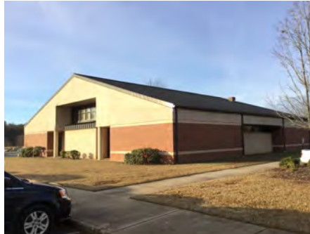
2). Northeast Elevation - Feb 12, 2017
