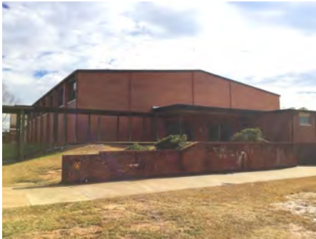
4). West Elevation - Feb 16, 2017
