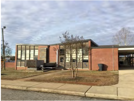
1). East Elevation - Feb 16, 2017
