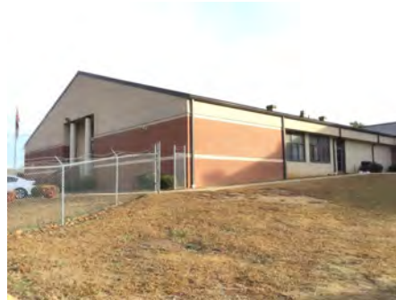
5). West Elevation - Feb 12, 2017
