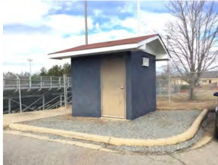
2). Southeast Elevation - Feb 15, 2017
