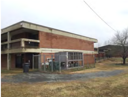
4). West Elevation - Feb 12, 2017
