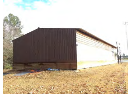
3). West Elevation - Feb 15, 2017
