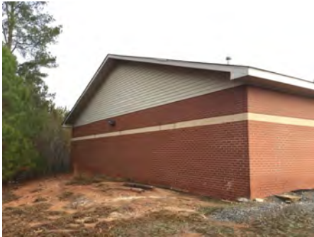
4). West Elevation - Feb 12, 2017
