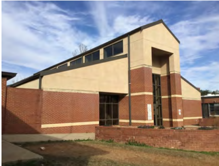
1). South Elevation - Feb 16, 2017
