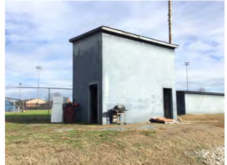
3). Southwest Elevation - Feb 15, 2017
