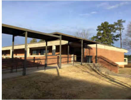
2). East Elevation - Feb 12, 2017
