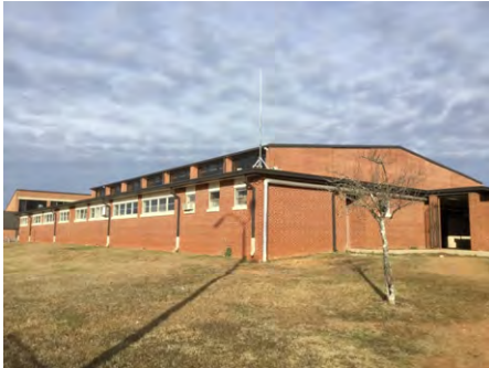
1). Southeast Elevation - Feb 16, 2017
