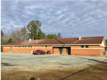
1). South Elevation - Feb 12, 2017
