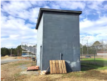
4). East Elevation - Feb 15, 2017
