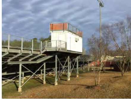
2). Southeast Elevation - Feb 12, 2017
