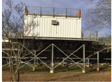
3). South Elevation - Feb 12, 2017
