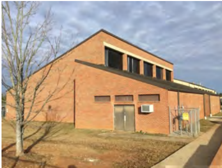
4). South Elevation - Feb 16, 2017
