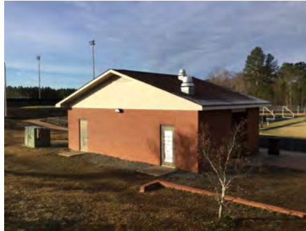
2). East Elevation - Feb 12, 2017
