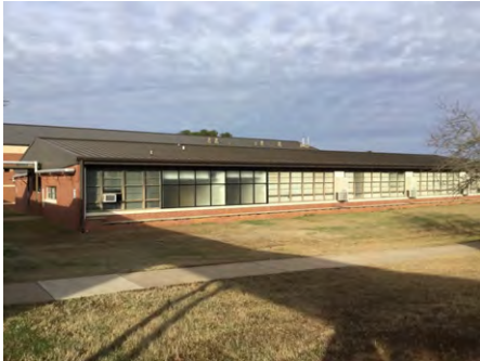
1). East Elevation - Feb 12, 2017
