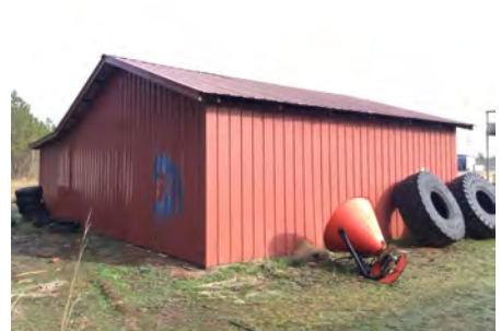
3). Southwest Elevation - Feb 12, 2017
