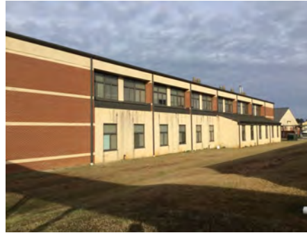
2). East Elevation - Feb 12, 2017
