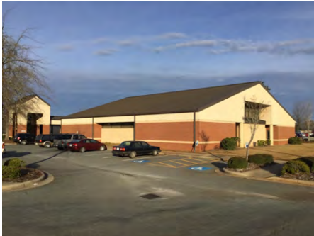
1). Southeast Elevation - Feb 12, 2017
