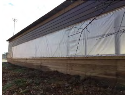
2). North Elevation - Feb 15, 2017
