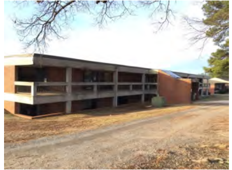
3). North Elevation - Feb 12, 2017
