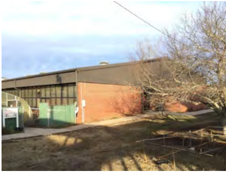
4). Southeast Elevation - Feb 12, 2017
