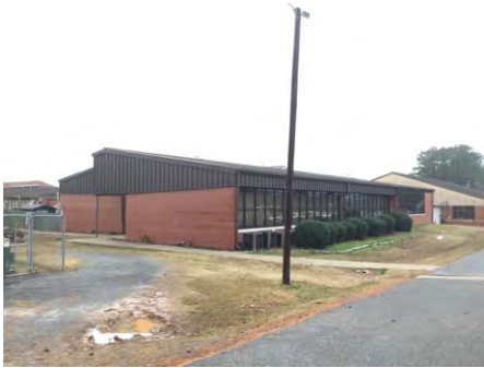
1). Northeast Elevation - Feb 12, 2017
