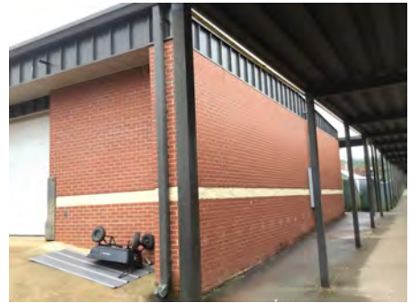
3). South Elevation - Feb 12, 2017
