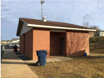
1). South Elevation - Feb 12, 2017
