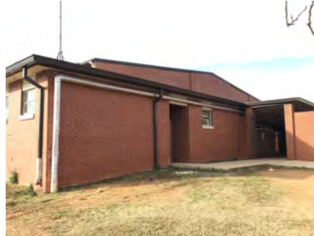
2). East Elevation - Feb 16, 2017
