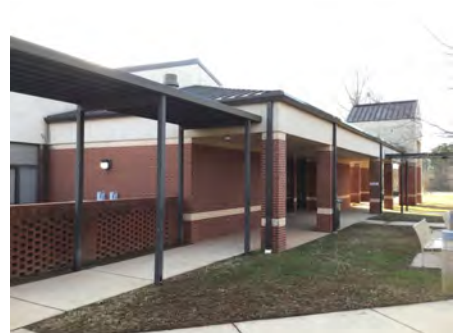
3). West Elevation - Feb 12, 2017
