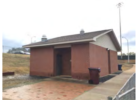
3). North Elevation - Feb 12, 2017
