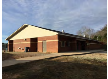
3). Northeast Elevation - Feb 12, 2017
