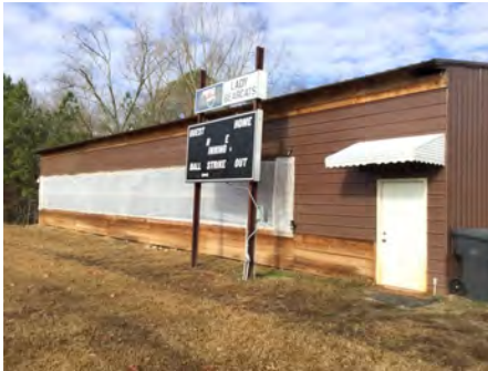
4). South Elevation - Feb 15, 2017
