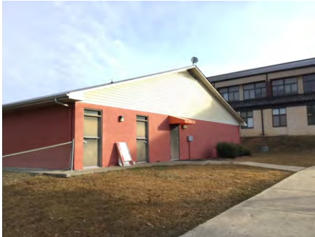
1). South Elevation - Feb 12, 2017
