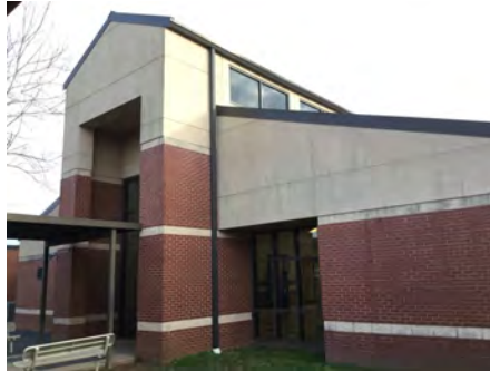
2). North Elevation - Feb 16, 2017
