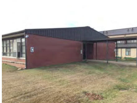
2). North Elevation - Feb 12, 2017
