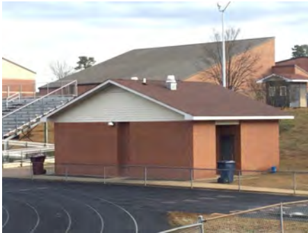
4). West Elevation - Feb 12, 2017
