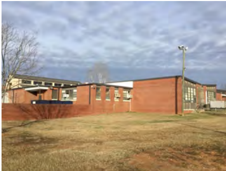
4). Southeast Elevation - Feb 16, 2017
