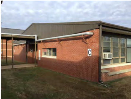
4). South Elevation - Feb 12, 2017
