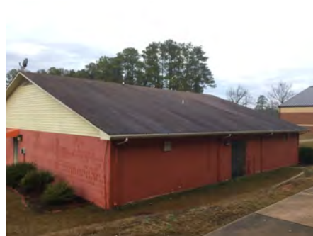
2). East Elevation - Feb 12, 2017
