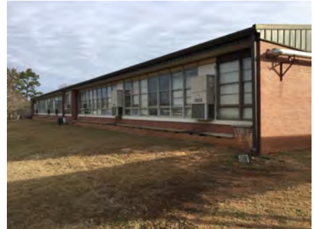
3). West Elevation - Feb 12, 2017
