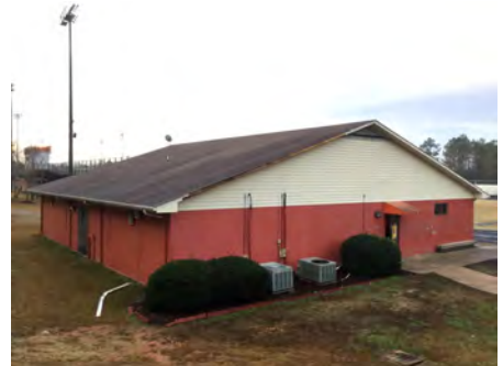
3). North Elevation - Feb 12, 2017
