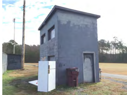
2). Northwest Elevation - Feb 15, 2017
