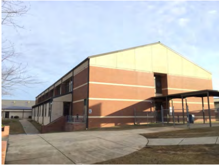
1). South Elevation - Feb 12, 2017
