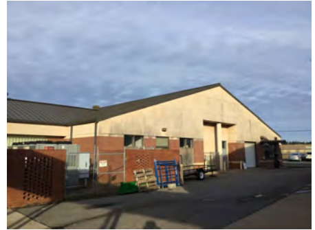
3). East Elevation - Feb 12, 2017
