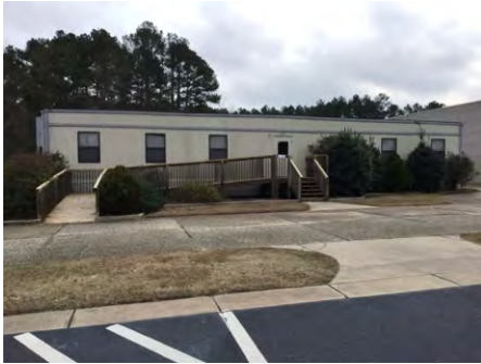
1). North Elevation - Jan 19, 2017
