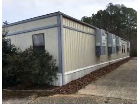
2). Northwest Elevation - Jan 19, 2017
