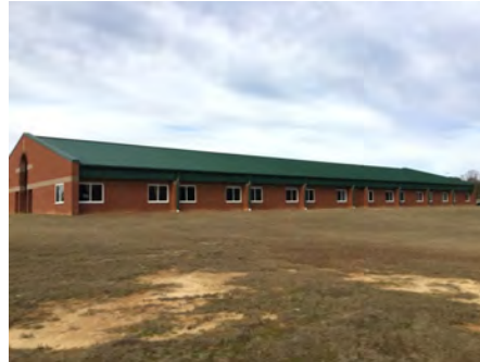
2). Southeast Elevation - Feb 08, 2017
