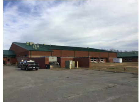
3). Southwest Elevation - Feb 08, 2017
