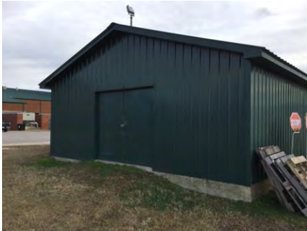
1). North Elevation - Jan 12, 2017
