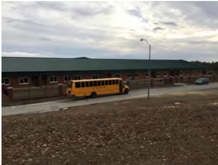
4). Northwest Elevation - Feb 08, 2017
