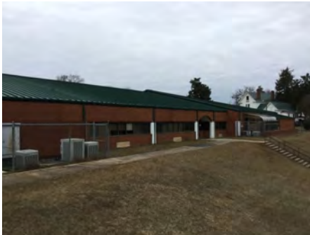
4). East Elevation - Mar 06, 2017
