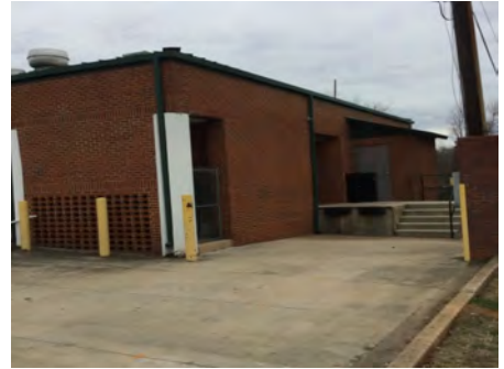
3). Southwest Elevation - Feb 10, 2017
