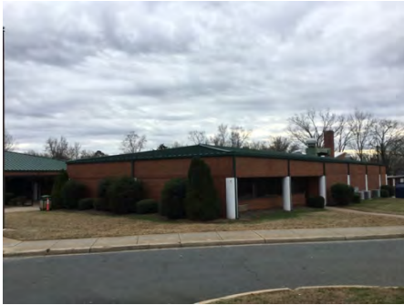
1). Northeast Elevations - Feb 10, 2017
