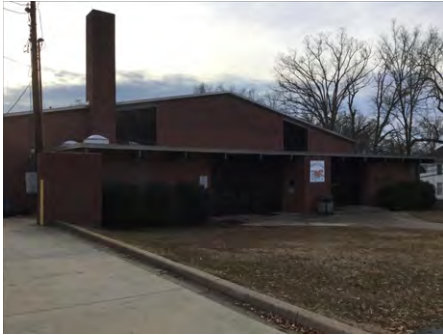
1). Northwest Elevation - Jan 20, 2017
