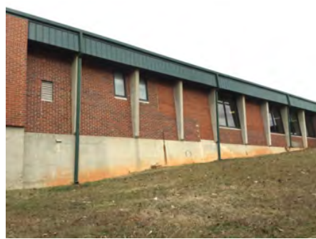
2). Southeast Elevation - Feb 10, 2017
