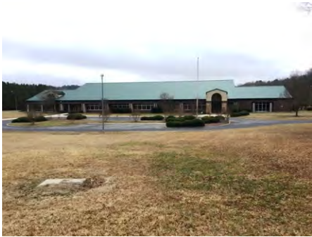
1). North Elevation - Jan 19, 2017
