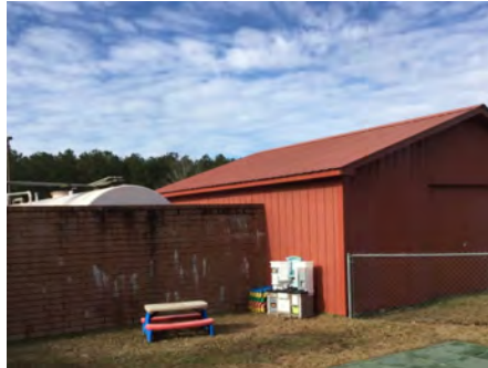
2). South Elevation - Mar 07, 2017
