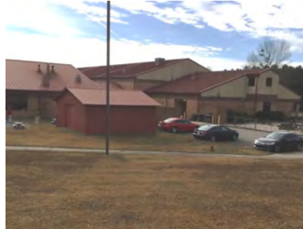
2). North Elevation - Jan 09, 2017
