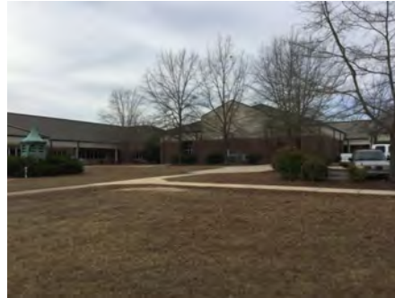
2). North Elevation - Feb 08, 2017
