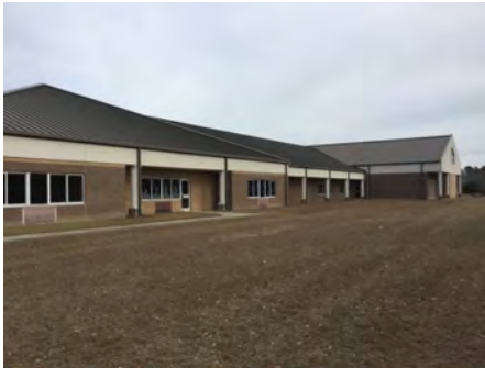
4). South Elevation - Feb 08, 2017
