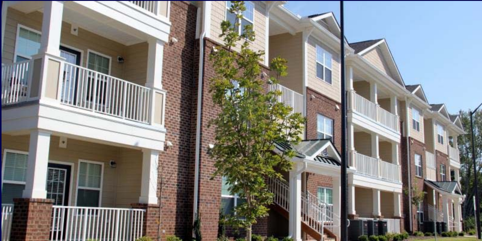
Low-Income Housing Tax Credit Project in Morganton, NC
