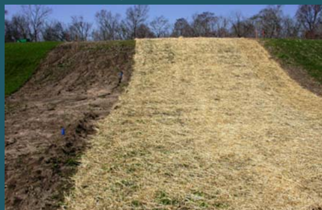
Surface stabilization protects soil by slowing water velocity and holding seed until vegetation can become established.
