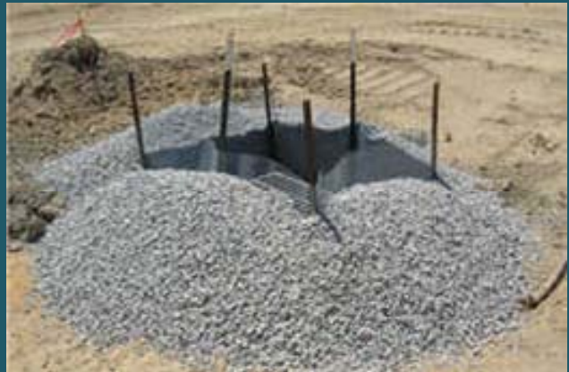
Inlet protection measures are intended to protect inlet points of runoff drainage.
