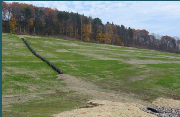
Temporary slope drains use flexible tubing or a conduit that extends from the top to the bottom of a cut or fill slope.
