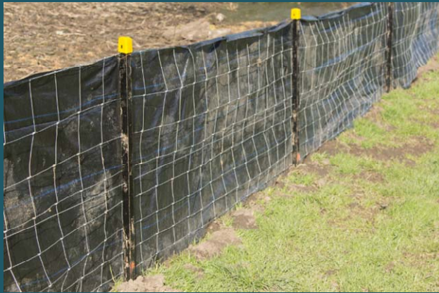
Silt fences are cloth barriers that stretch along disturbed areas and capture sediment from the flow of water.
