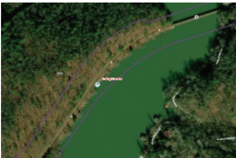
Eroding Shoreline – West of Lake Summit Bridge (35.23, -82.40) Shoreline along track eroding into lake, potentially undermining rail bed.
