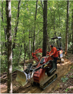
Contractors working on Jim Branch Trail
