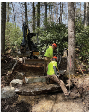
Trail contractor installing steps along Grassy Creek Falls Trail
