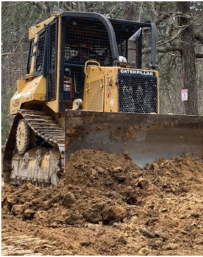
DSRF staff grading for the overflow parking area
