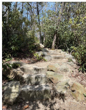
Finished steps on Grassy Creek Falls Trail
