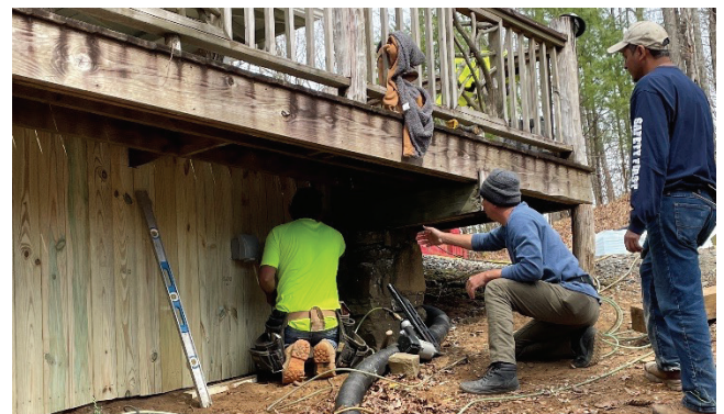
Contractors enclosing the lower level of the law enforcement cabin
