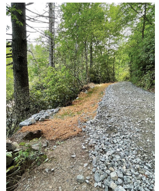
Triple Falls Trail added an improved walking surface and erosion control measures.
