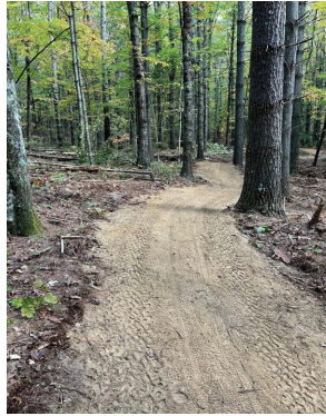
Hooker Creek Trail repairs completed
