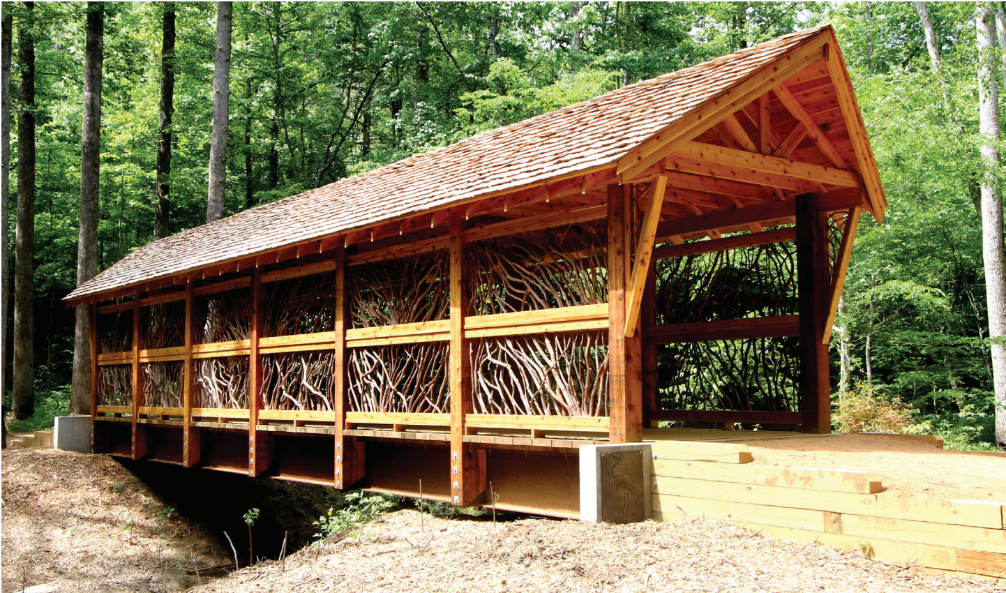
Bridge on the Fonta Flora State Trail
