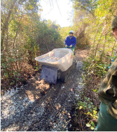
CCNC crews used motorized buggies to deliver gravel to trails at Jones Lake State Park
