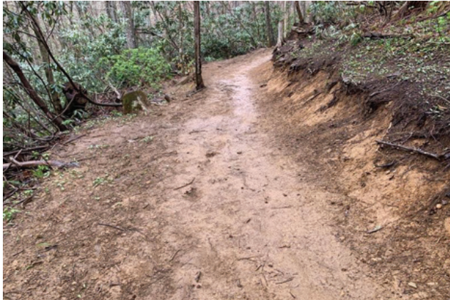
Widened and compacted trail tread on Profile Trail, Grandfather Mountain State Park
