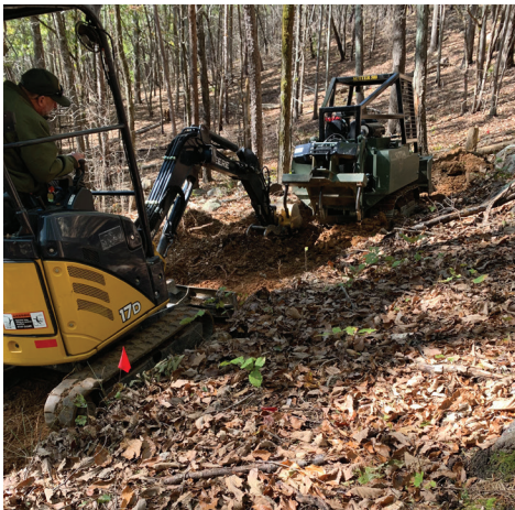
Workshop using mini-excavator and Trail Dozer at Crowders Mountain State Park
